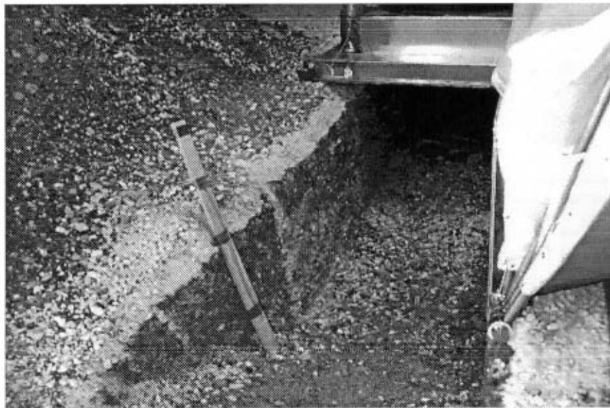
Figure 6. X2 Release Point Location — Sloped End of Trench, Spoil Side
