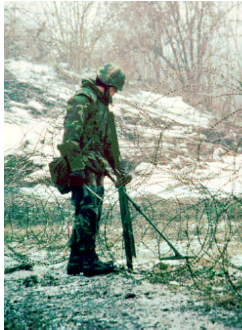
GI Searching for Mines in Bosnia, 1996 -Mine detection capabilities and equipment available to soldiers in the field have changed little in 50 years. Note the probe rod in this soldier's right hand.
