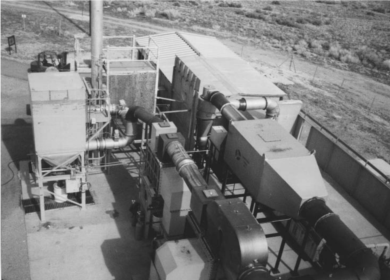
FIGURE 8: OVERVIEW OF DEACTIVATION FURNACE SYSTEM
