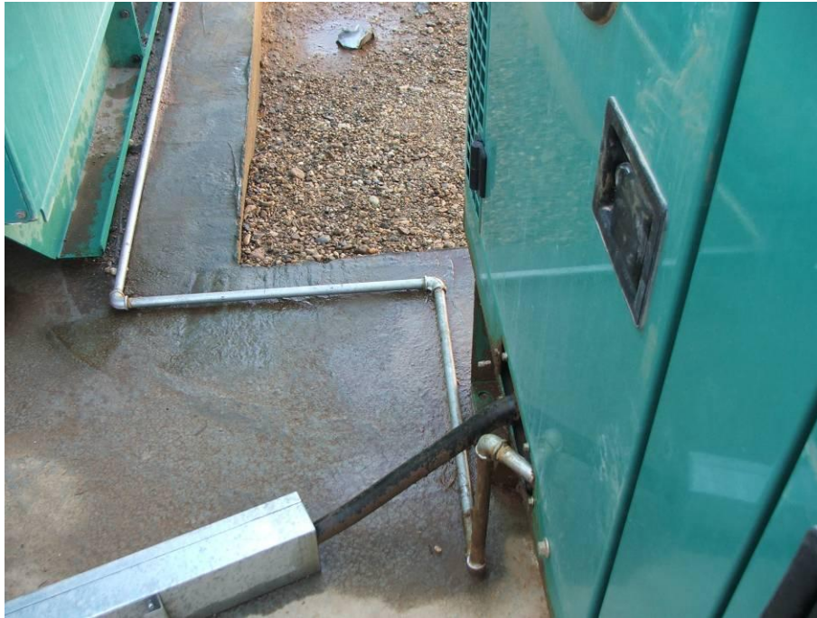
Site Photo 17. Diesel fuel spill and electrical line not installed correctly.
