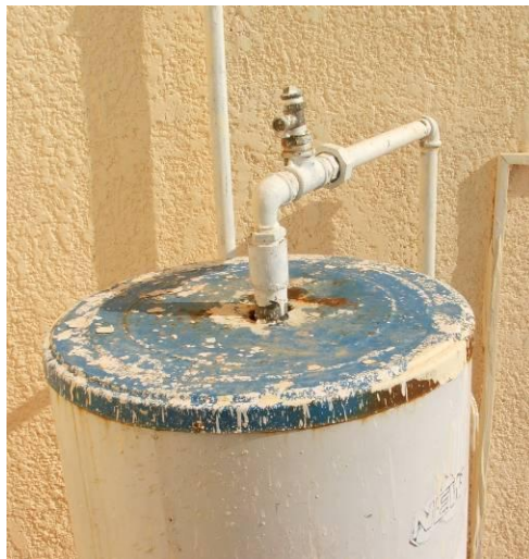
Site Photos 20 and 21. Non-functioning and possibly used hot water heaters
