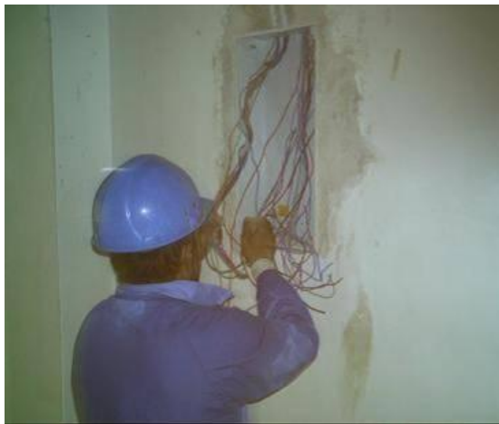
Site Photos 6 and 7. Installation of electrical wiring and mosaic tile, respectively (Courtesy of GRC)
