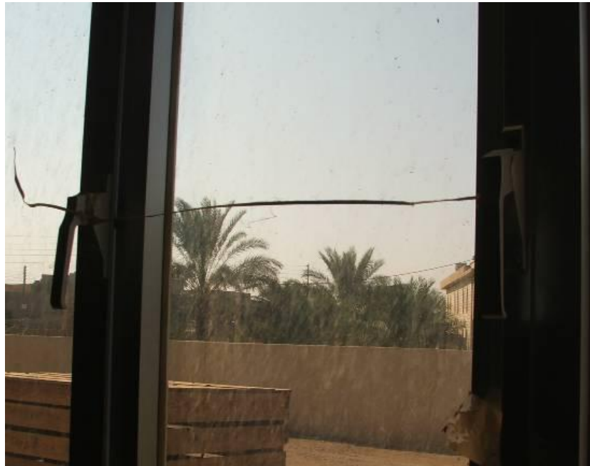
Site Photo 26. Poorly constructed and unsecured window.
