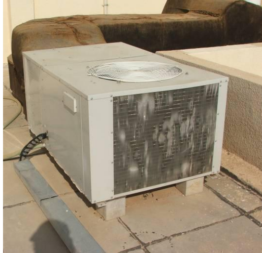
Site Photo 27. HVAC unit non-functioning and damaged
