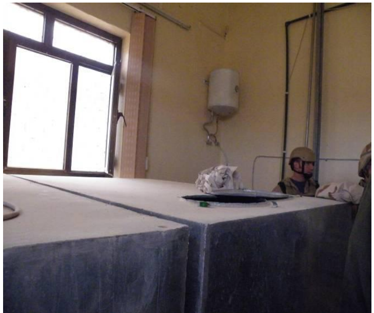
Site Photo 7. Uncovered equilization tank
