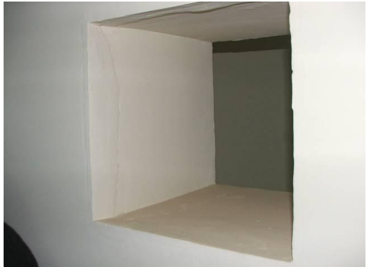
Site Photo 11. Missing observation window
