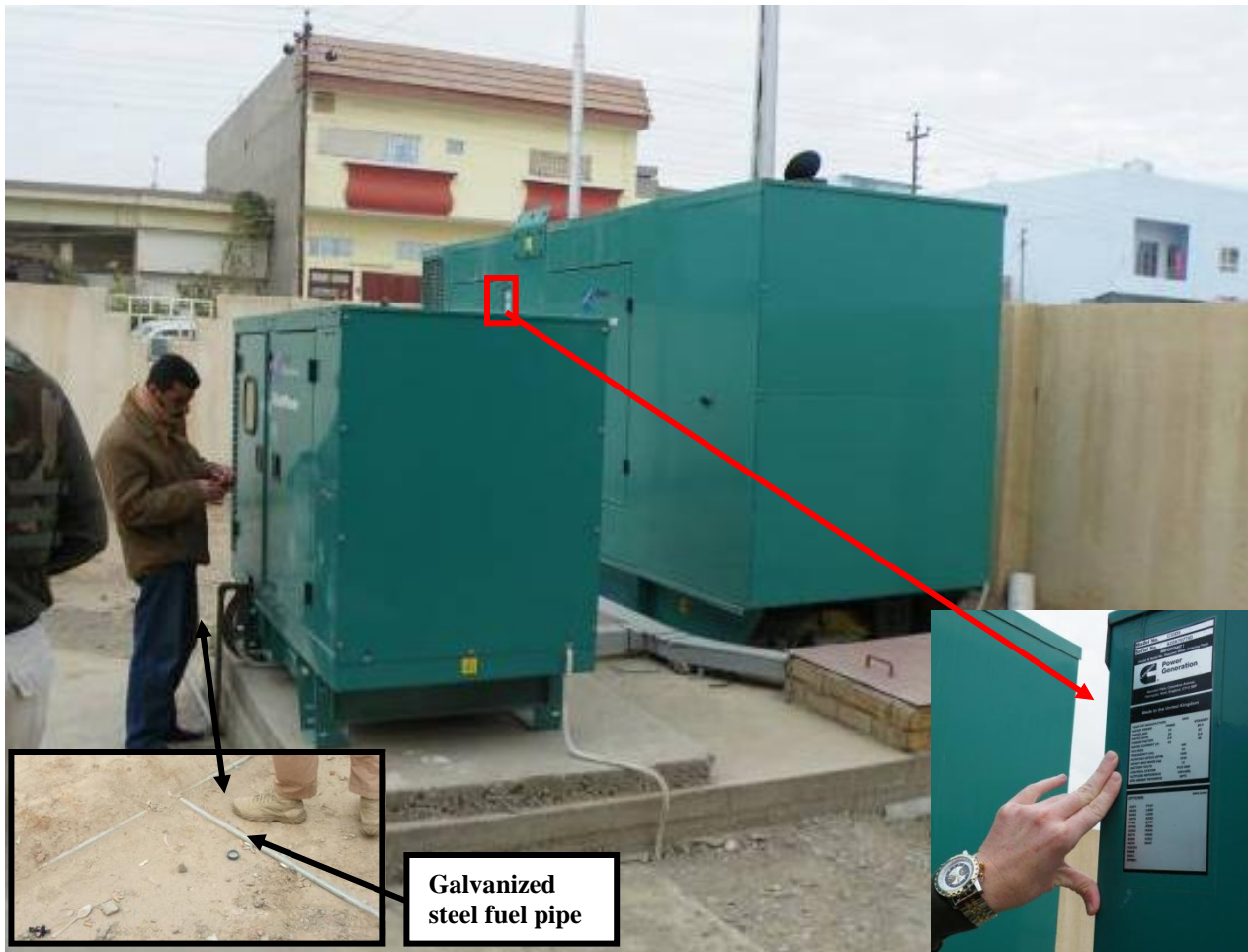
Site Photo 4. Two generators providing primary and emergency backup power for the PHC
