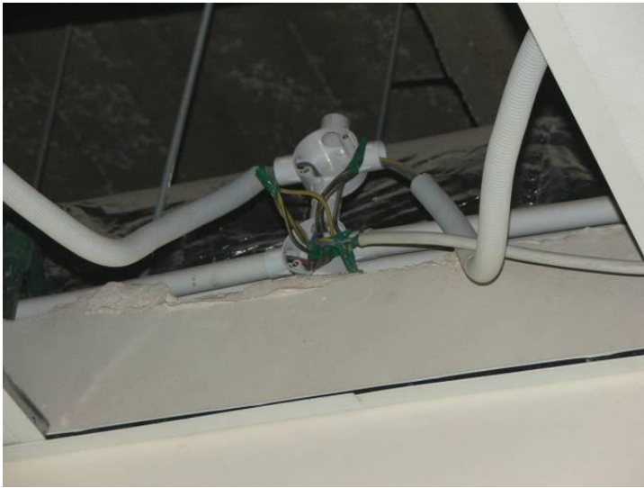
Site Photo 15. Poor electrical connection
