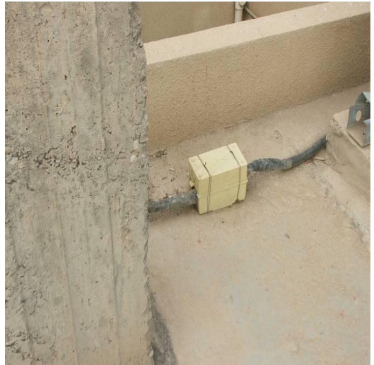
Site Photo 13. Makeshift electrical junction
