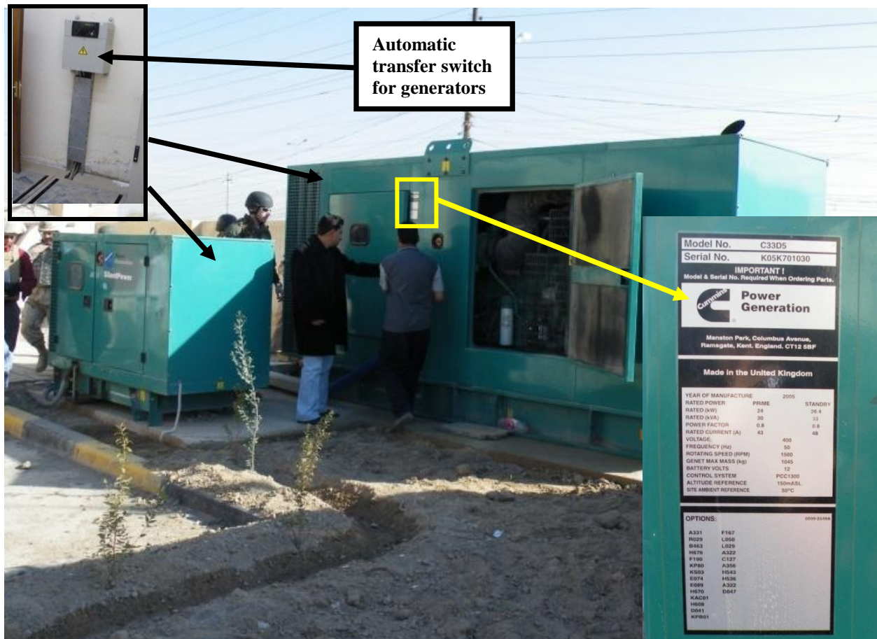
Site Photo 5. Two generators providing primary and emergency backup power for the PHC
