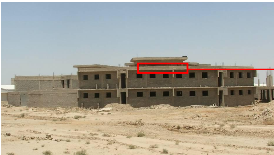
Site Photo 10. Medium security building that structural assessment recommended replacing
