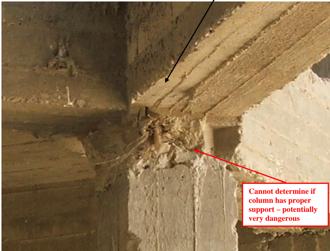
Site Photo 18. Close-up of Site Photo 17
