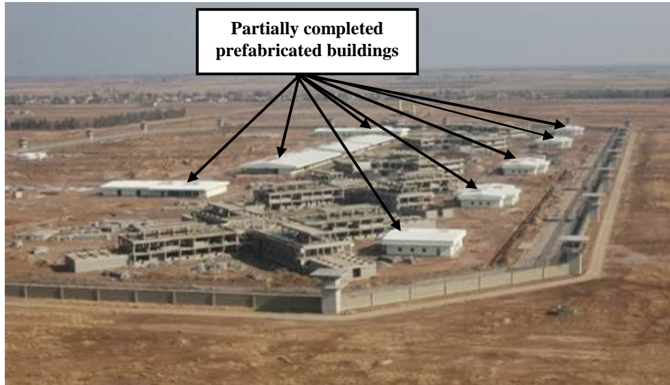
Site Photo 25. Aerial view of KBS Correctional Facility (Courtesy of the USACE)
