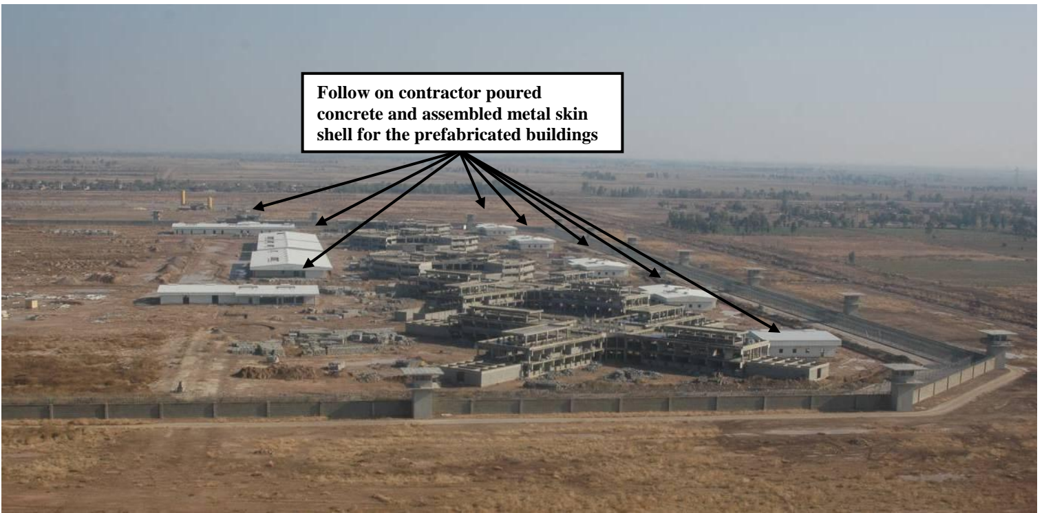
Site Photo 4. Status of construction at the time of the follow-on contractor’s termination (Courtesy of the USACE)
