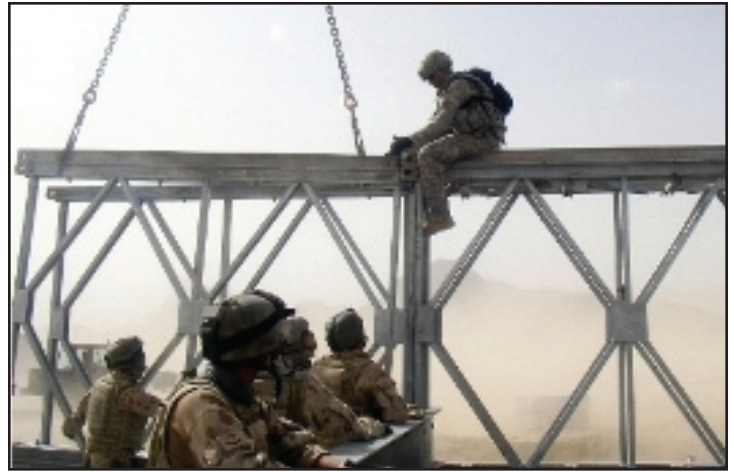
Australian and American Army combat engineers work together to build a replacement bridge in Afghanistan. (U.S. Army photo)
