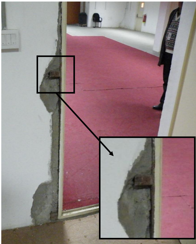
Site Photo 9. Interior door damage
