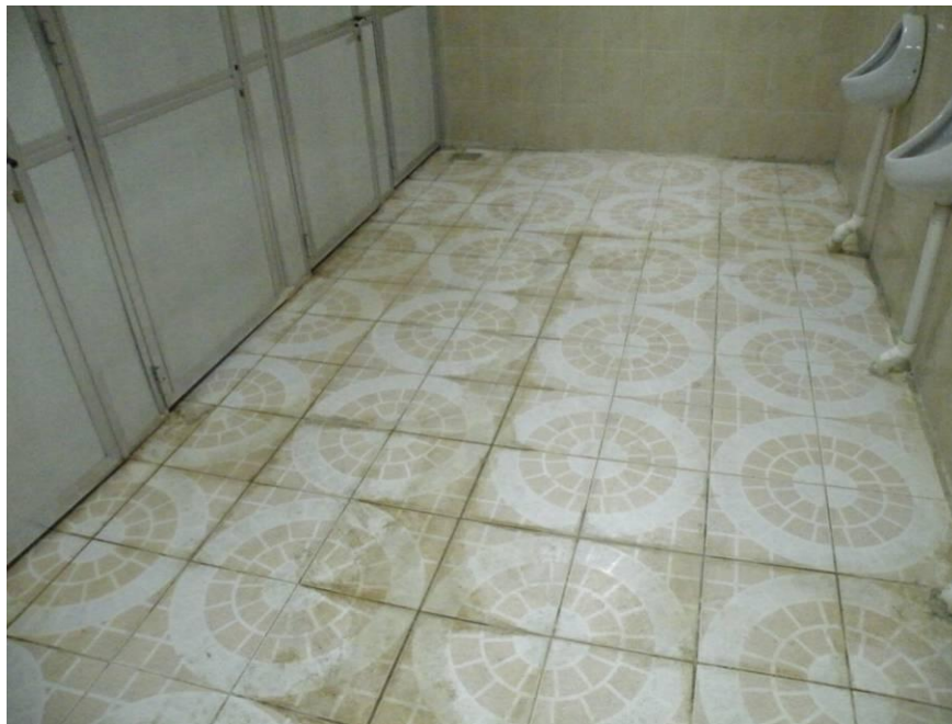
Site Photo 15. Contractor replaced previously cracked and buckling floor tiles (See Site Photo 8 for original condition of bathroom floor.)
