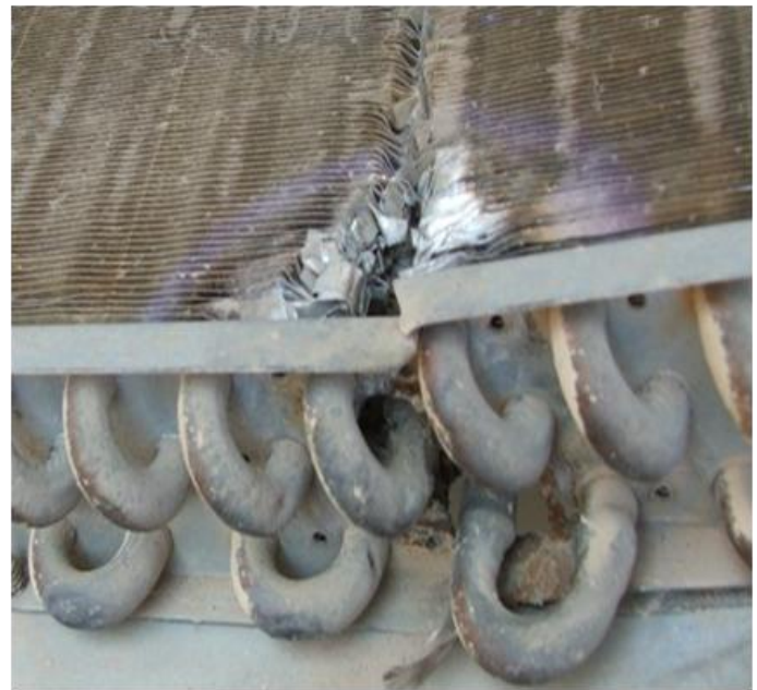
Site Photos 11 and 12. Soldering done on HVAC units
