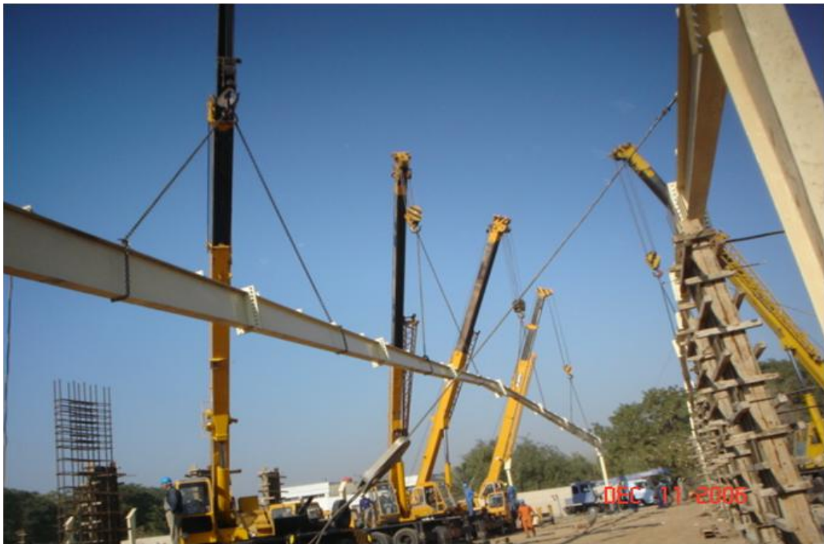
Site Photo 1. Initial construction of the steel columns prior to the structural failure (Courtesy of GRC)
