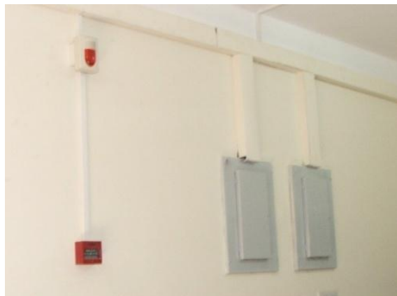
Site Photos 7 and 8. Installation of new wire molding, outlets, light fixtures and new main distribution panels (left) and careless over-painting of intercom system (right).
