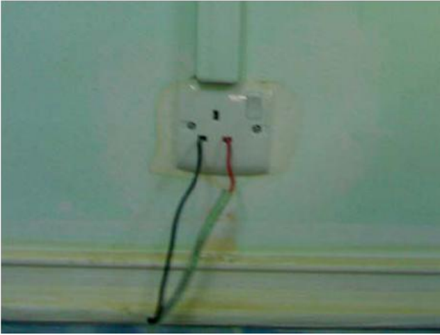
Site Photos 14 and 15. Unsafe electrical practices used by the contractor and captured in daily QA reports (Courtesy of USACE)
