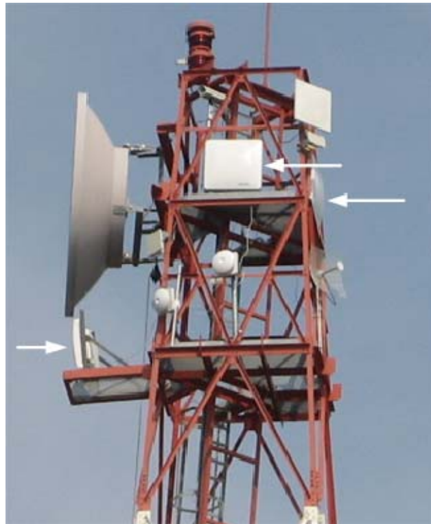
Figure 11. Phased array antennas mounted on Comms Tower on Ao Manao Airbase in Thailand.
