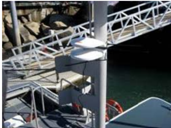
Figure 6. Ruckus device mounted to mast of USCG UTB.
