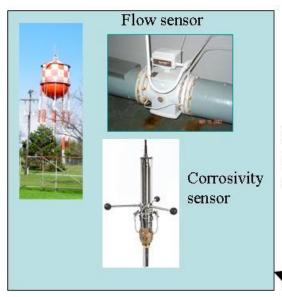
Water system outfitted with sensors and RTUs
