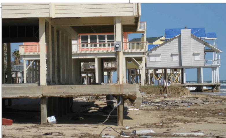
Figure 5 (right). Undermining of concrete slabs of beach residences on west Galveston Island.
