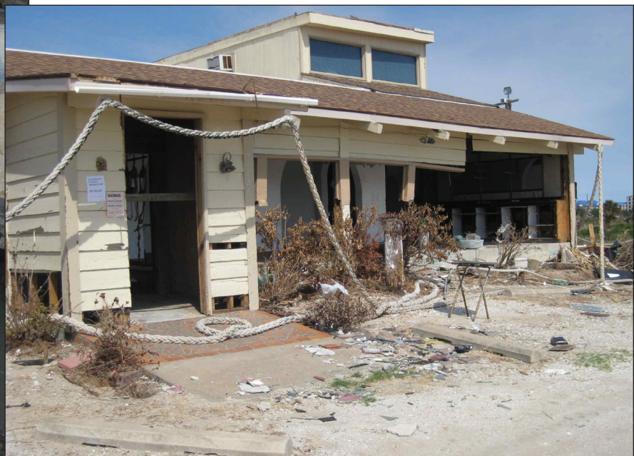
Figure 8 (below). Flood damage by surge on structure facing the Gulf of Mexico, but more than 1,500 ft (450 m) from the beach.
