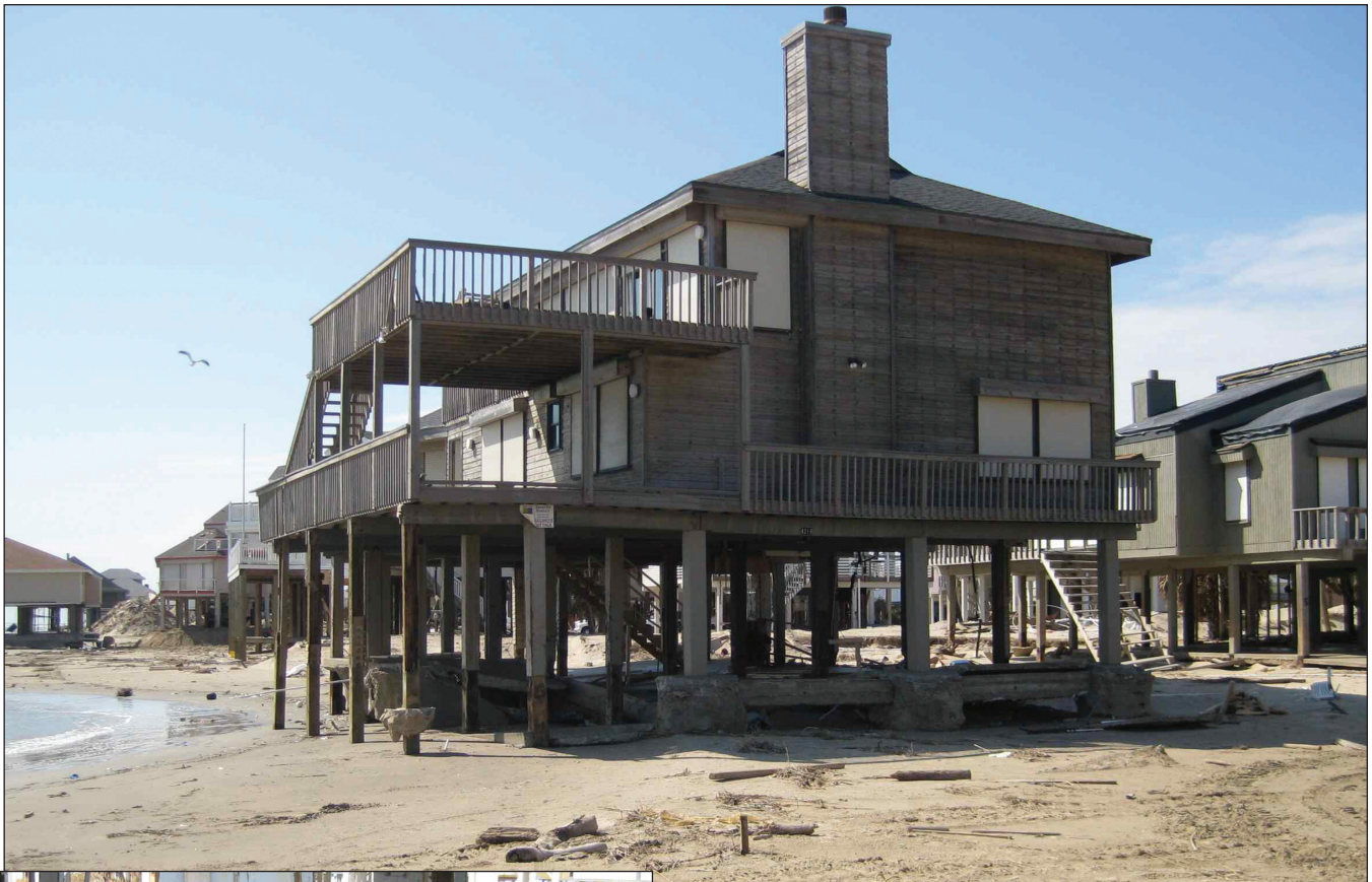
Figure 6 (above). Undermining of concrete slabs was progressively less with distance landward (to right of picture).
