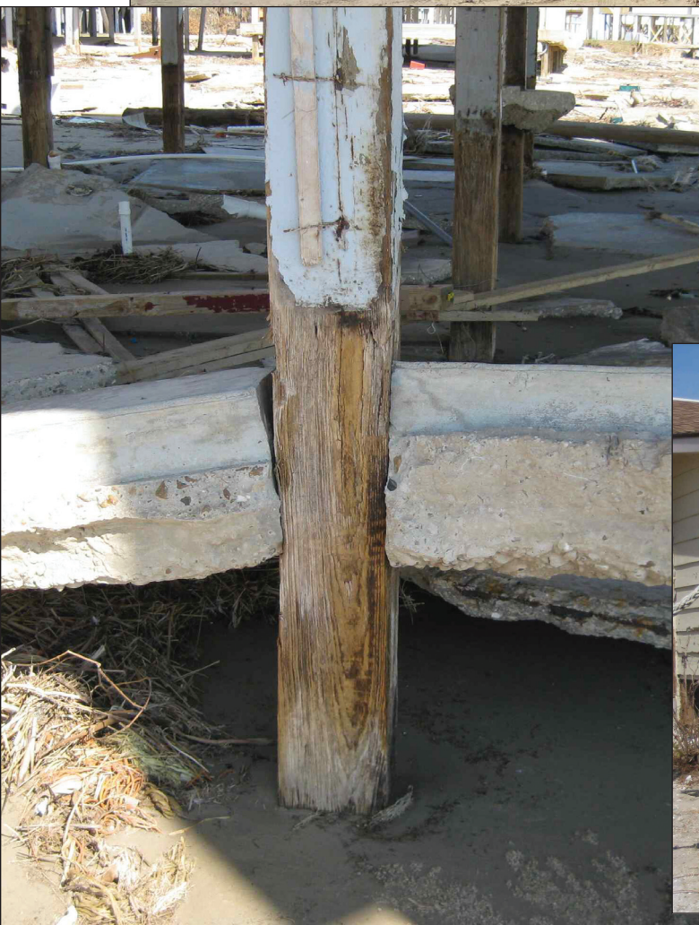
Figure 6 (above). Undermining of concrete slabs was progressively less with distance landward (to right of picture).
