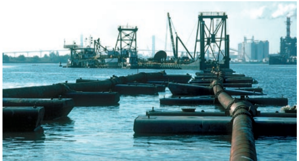
Figure 2. Dredging to maintain navigable depths at Savannah.
