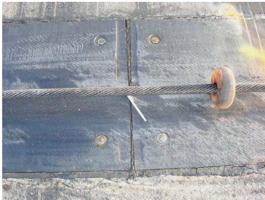
Figure 45. Condition of asphalt, sealant, and panels on Runway 22 at Holloman AFB.
