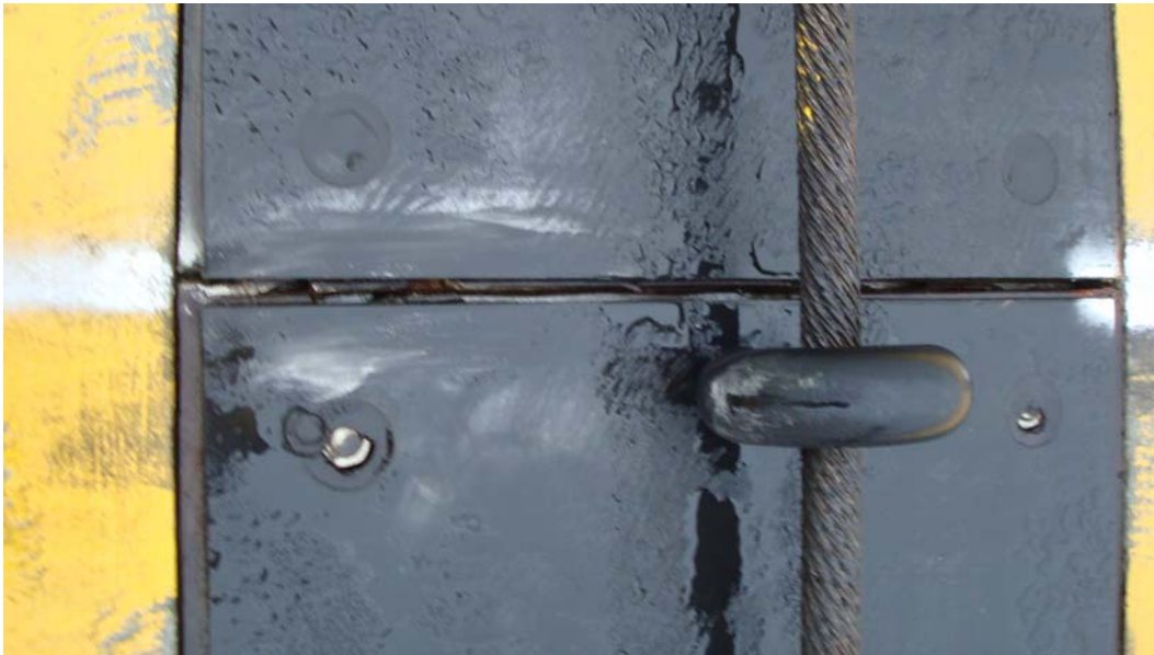
Figure 68. Loss of sealant in recess for anchor at Runway 22 R at Shaw AFB.
