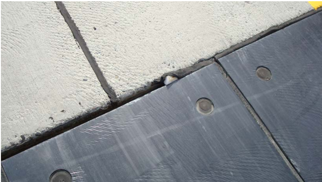
Figure 30. Minor surface wear of the pavement surface and rounding of the edges on Runway 06 at Elmendorf AFB.
