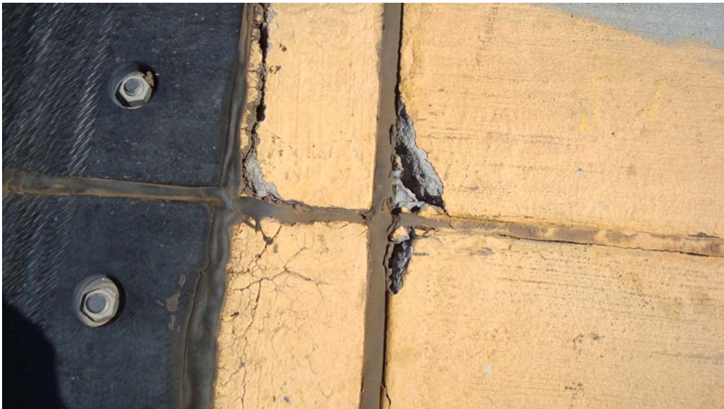
Figure 55. Some localized spalling of concrete at Luke AFB.
