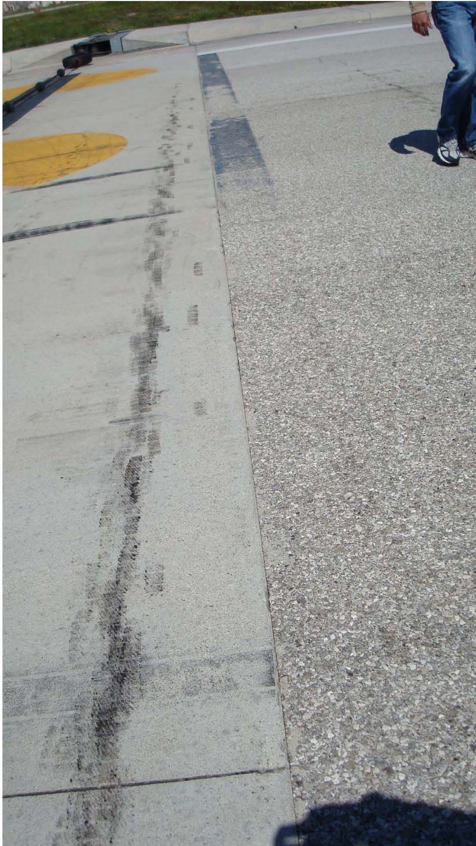
Figure 5. SMA mixture placed adjacent to concrete foundation for barrier panels at Aviano AB.
