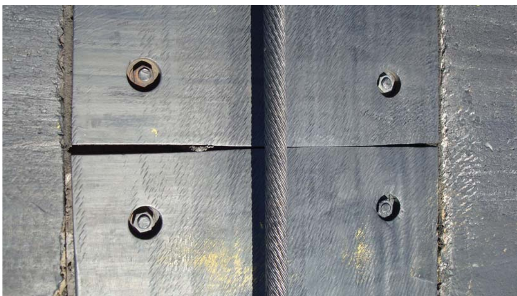
Figure 15. Variable width of joints in polyethylene panels at Davis-Monthan AFB.
