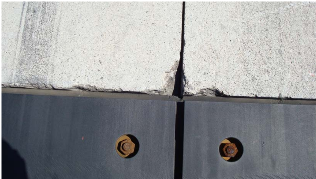
Figure 9. Some spalling of concrete adjacent to panels and at contraction joint at Aviano AB.
