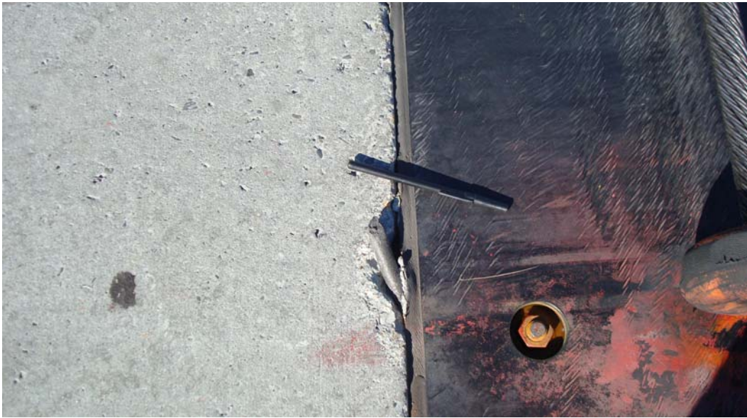
Figure 21. Exposure of backer rod between panels and concrete pavement (south end of runway) at Eielson AFB.
