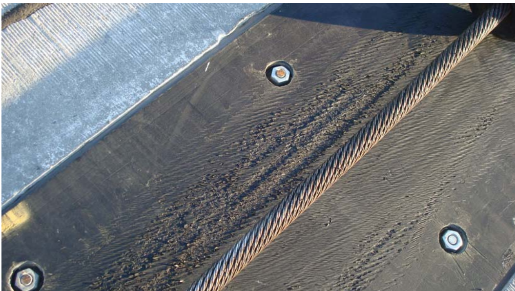
Figure 88. Barrier Cable at Tyndall Runway 13 L showing minor damage to panel from beating of the cable.
