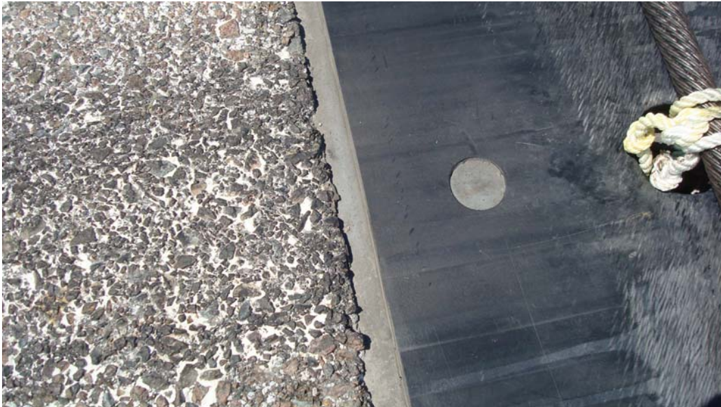
Figure 59. Condition of sealant after 3 months in place at MacDill AFB.
