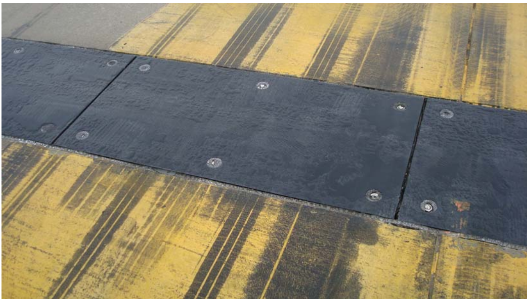
Figure 74. Offset of joint between panels and joint in concrete at Runway 22 L at Shaw AFB.
