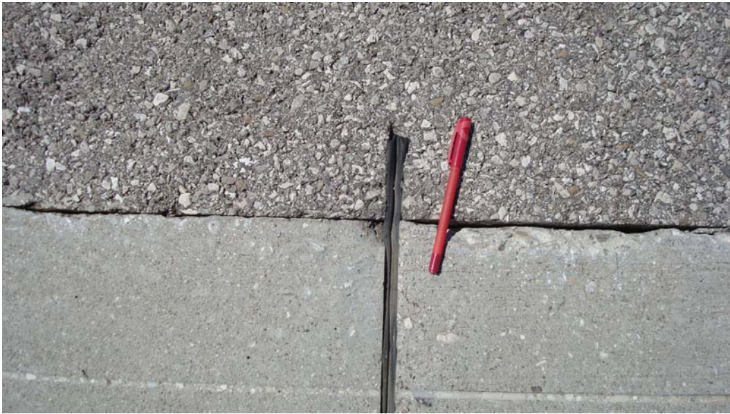
Figure 6. No damage of the SMA and slight spalling of the concrete slab at Aviano AB.
