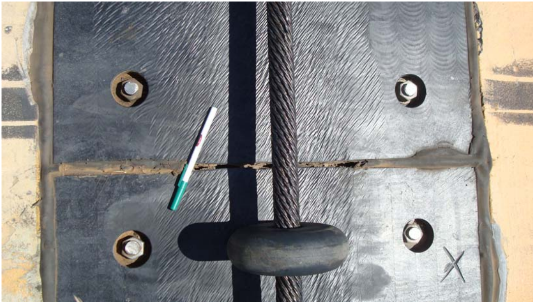
Figure 56. Condition of sealer satisfactory in spots and damaged in other areas at Luke AFB.
