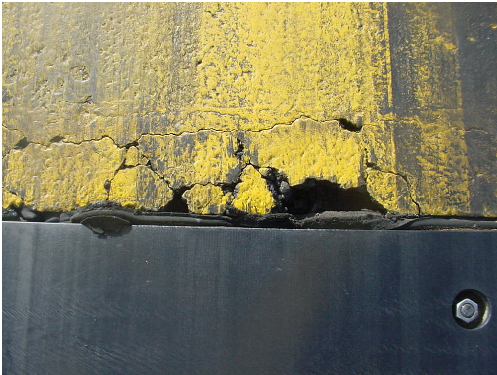
Figure 62. Loss of asphalt mixture immediately adjacent to the panels at McChord AFB.
