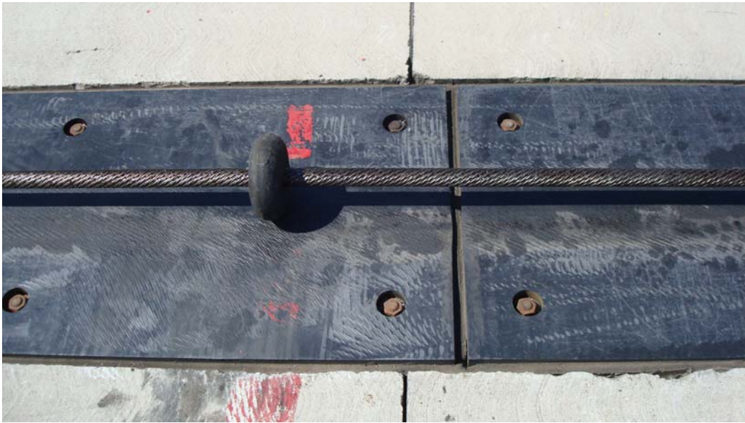
Figure 10. Anchors for panels placed very close to contraction joint in concrete at Aviano AB.
