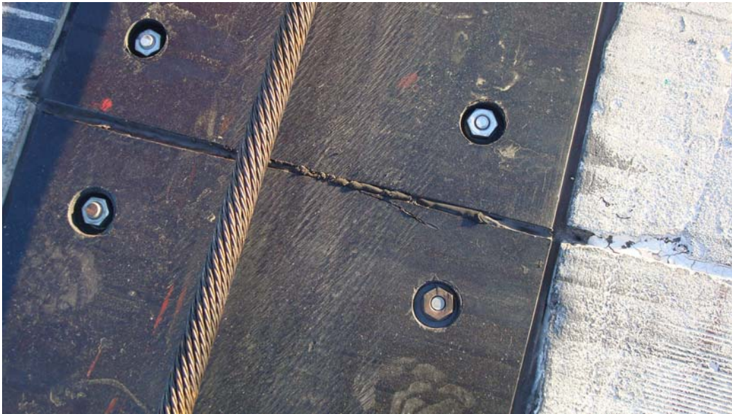
Figure 86. Barrier cable at Runway 13 L at Tyndall AFB showing no sealant in anchor recess.
