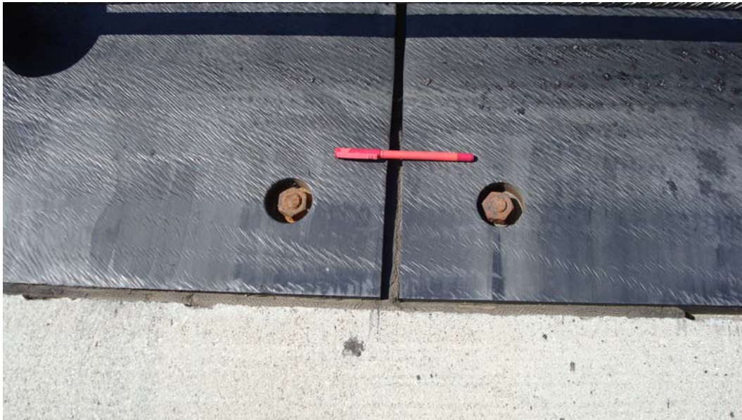
Figure 8. Sealant in poor shape adjacent to panels at Aviano AB.
