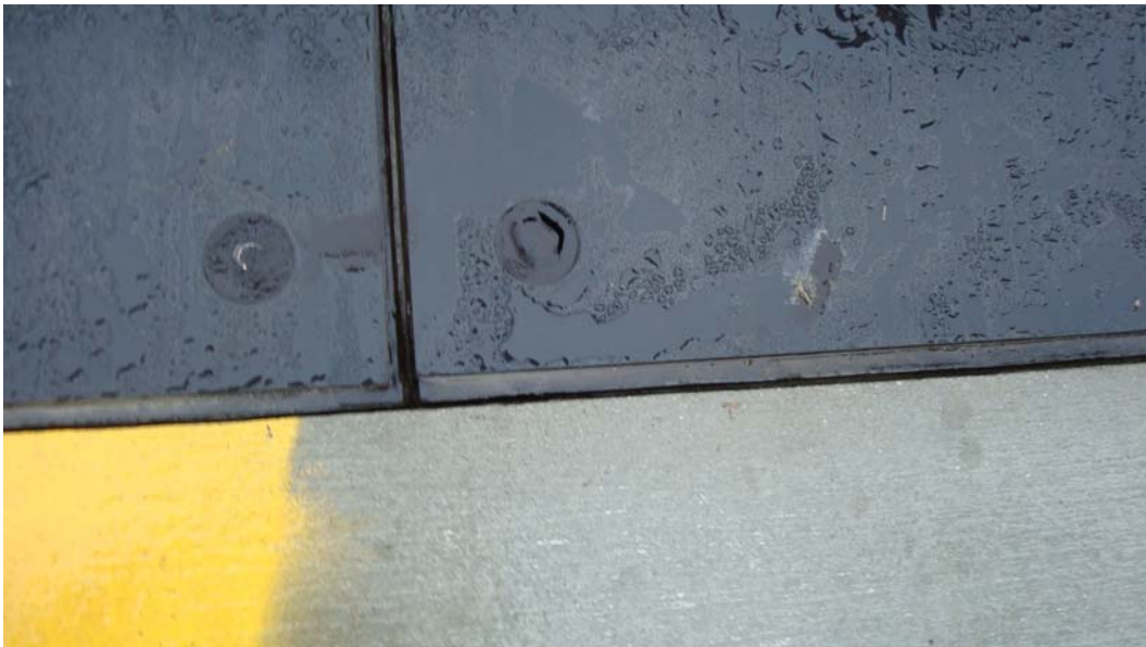
Figure 67. Performance of sealant at Runway 22 R at Shaw AFB.
