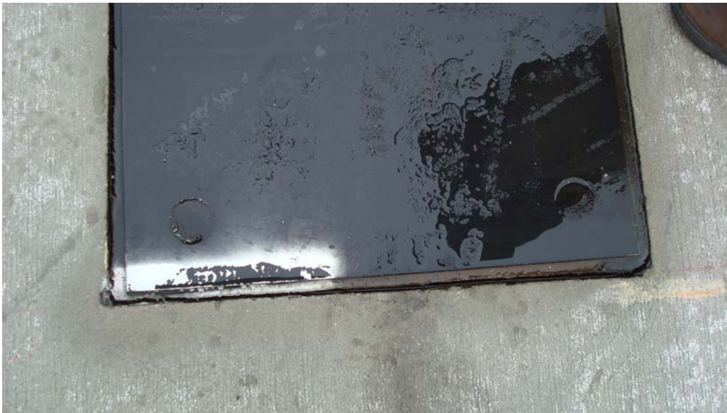
Figure 70. Sealant pulled away from concrete at Runway 4 R at Shaw AFB.
