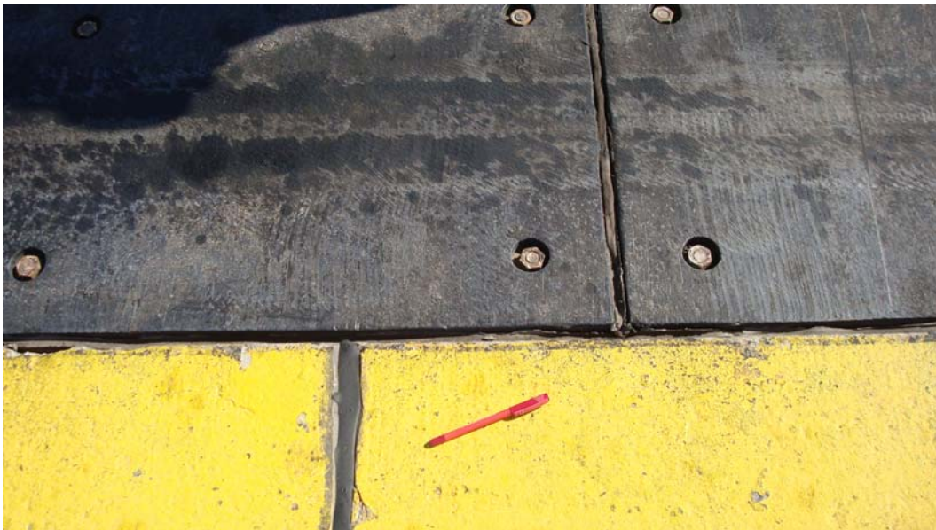
Figure 82. Joints between panels did not match joints in adjacent concrete at Spangdahlem AFB.
