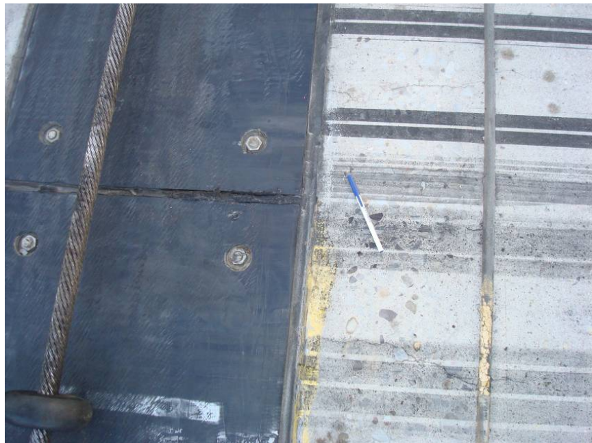
Figure 41. Condition of panels, sealant, and concrete on Runway 34 at Holloman AFB.
