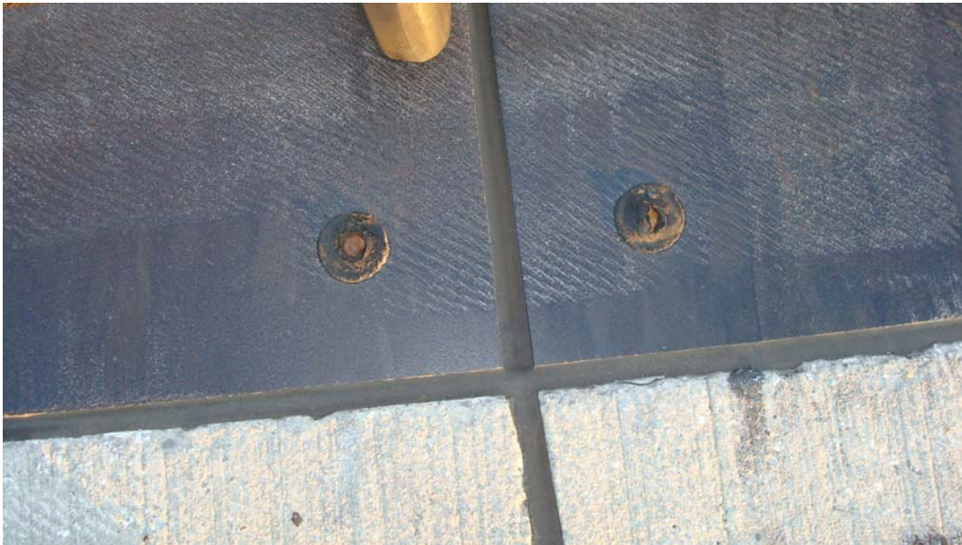
Figure 92. Barrier cable (BAK-12) at Runway 31 L at Tyndall AFB showing good sealant.
