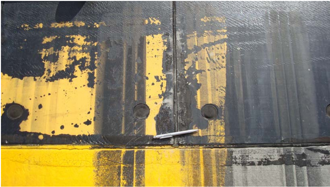
Figure 31. Sealant in reasonably good condition on Runway 06 at Elmendorf AFB.
