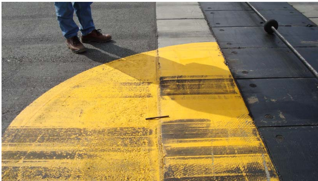
Figure 34. Bump between asphalt pavement and concrete strip on Runway 24 at Elmendorf AFB.
