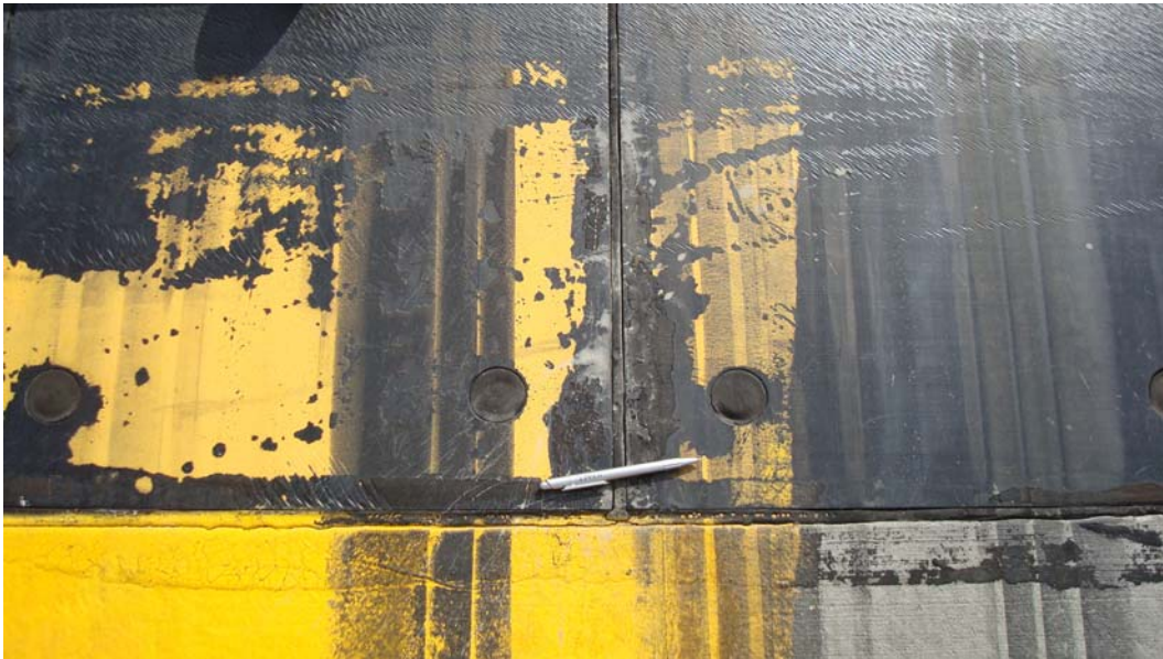
Figure 26. Condition of joint sealant on Runway 34 at Elmendorf AFB.
