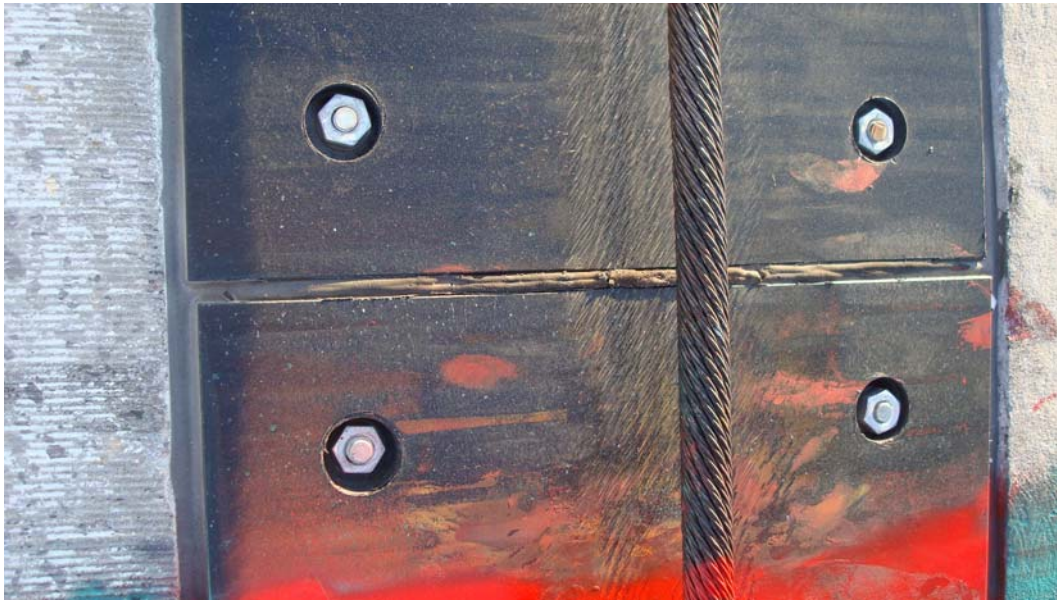
Figure 100. Loss of sealant effectiveness at joint between panels at Runway 13 R at Tyndall AFB.
