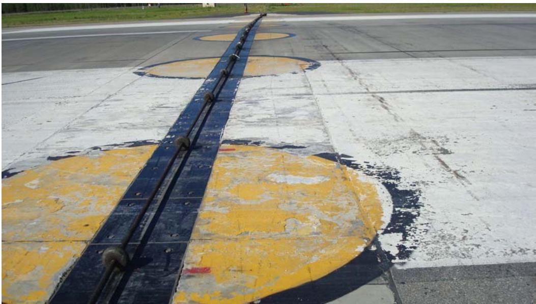
Figure 22. Overview of UHMW polyethylene panels at Eielson AFB showing concrete on both sides of the panels (north end of runway).
