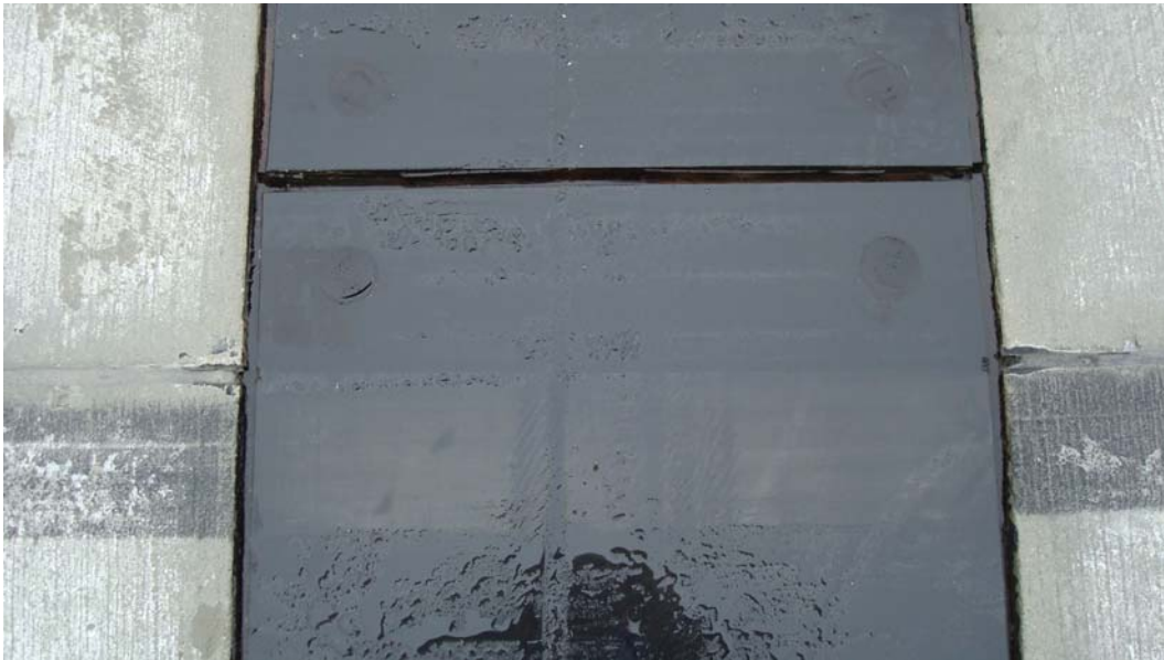
Figure 71. Joint in panels does not match joint in concrete at Runway 4 R at Shaw AFB.
