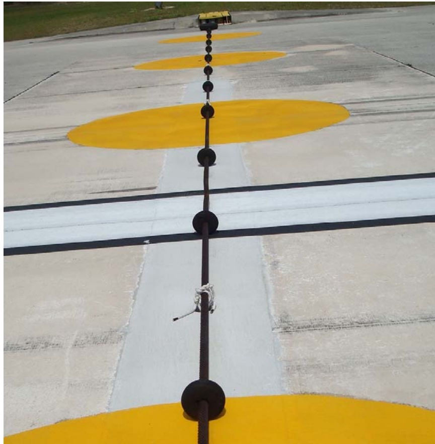
Figure 2. Typical patch area underneath cable in concrete pavement.
