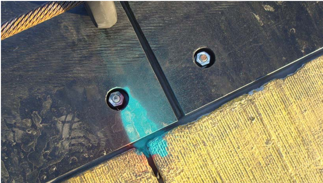
Figure 87. Barrier Cable at Runway 13 L at Tyndall AFB showing joints in concrete not matching joints between panels.
