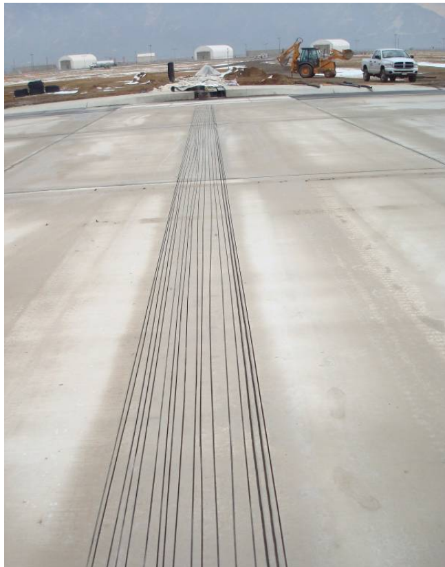
Figure 39. Saw cuts prior to removal of concrete for replacement of polyethylene panels on Runway 14 at Hill AFB.
