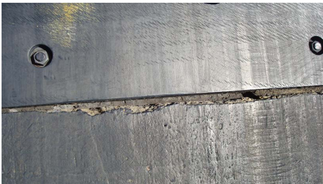
Figure 16. Condition of joint between concrete and polyethylene panel at Davis-Monthan AFB.
