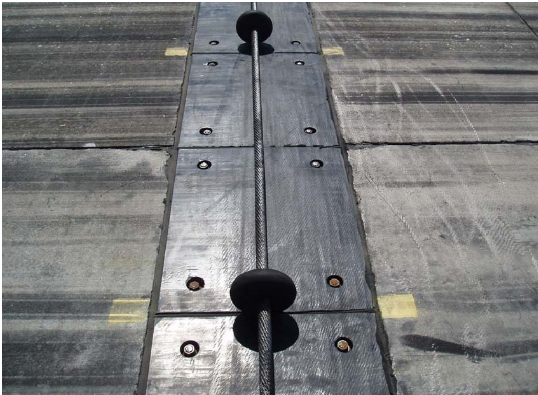
Figure 12. Condition of sealant around UHMW polyethylene panels at Buckley AFB.
