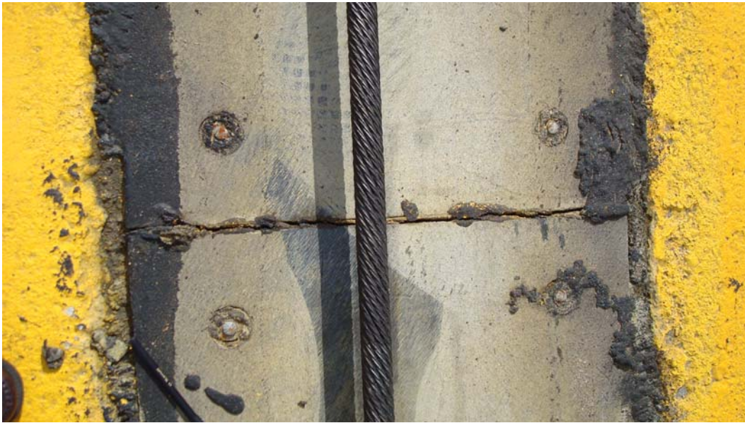
Figure 28. Partially sealed anchors on Runway 34 at Elmendorf AFB.
