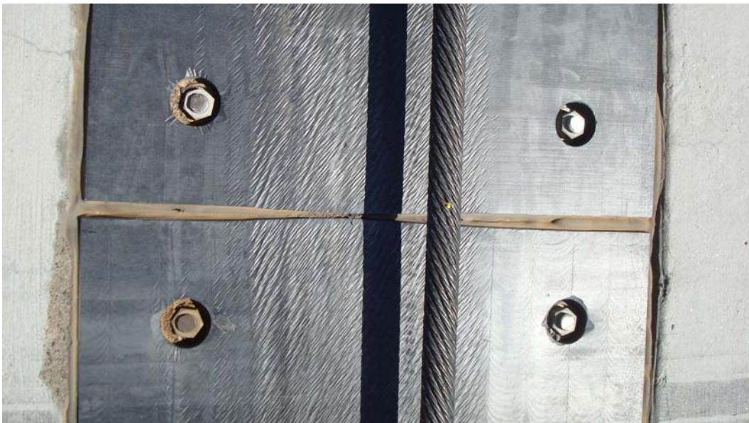
Figure 57. Some deformation in the panels and some wear from beating of the cable at Luke AFB.
