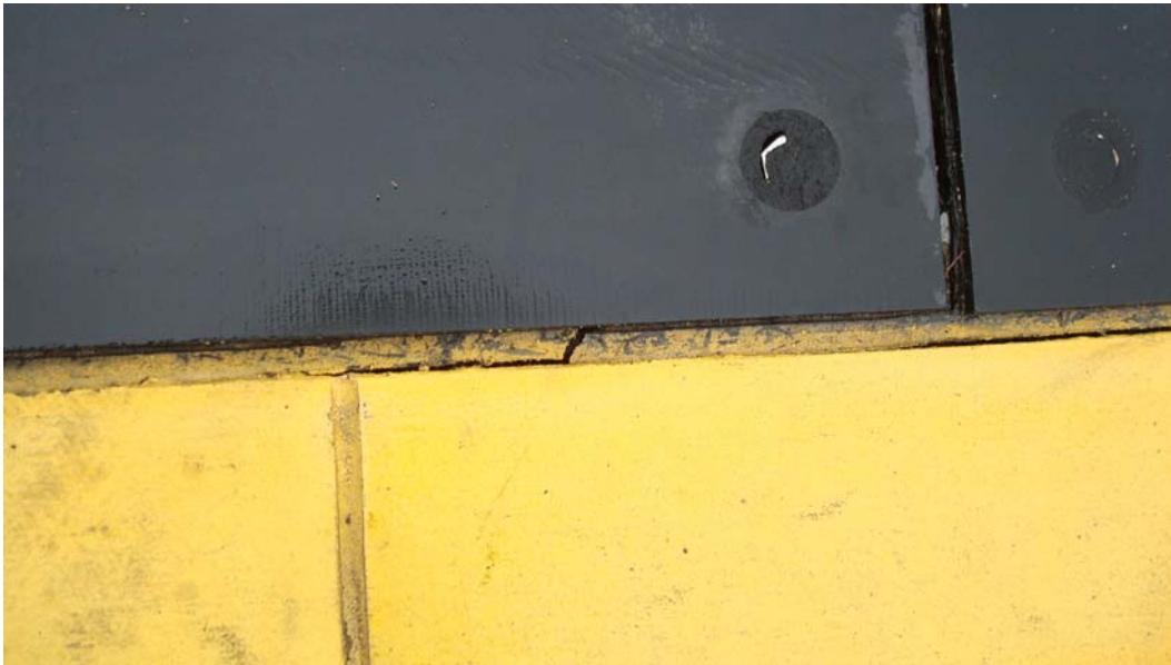
Figure 77. Joints in concrete do not match joints between panels at Runway 4 L at Shaw AFB.
