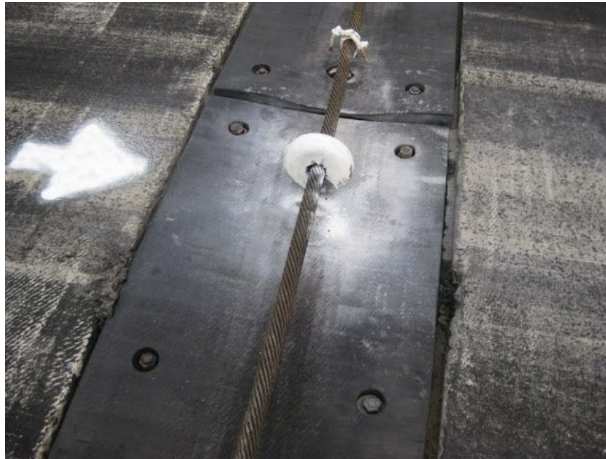
Figure 64. Deformed panels at Seymour Johnson AFB.
