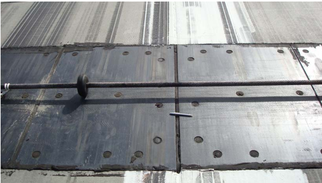
Figure 32. Sealant in poor condition on Runway 06 at Elmendorf AFB.
