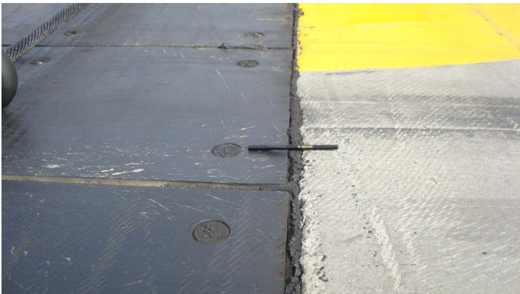
Figure 36. Poor performance of sealer between two adjacent panels and between the panels and the adjacent concrete on Runway 24 at Elmendorf AFB.
