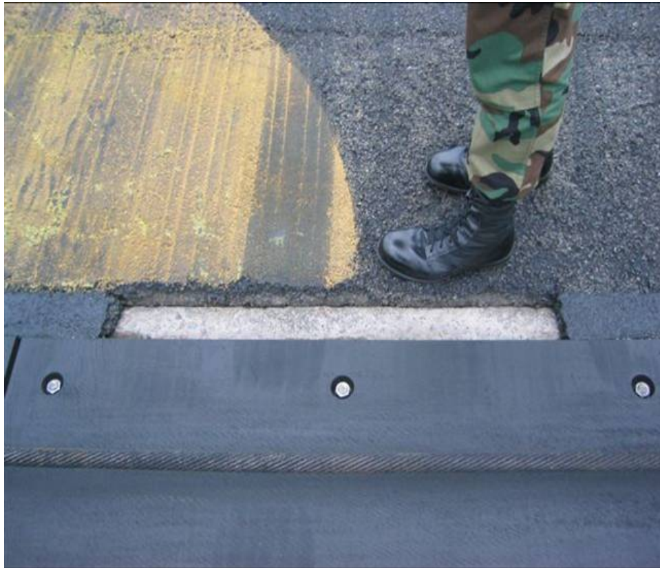
Figure 101. Remove damaged material and square up hole.
