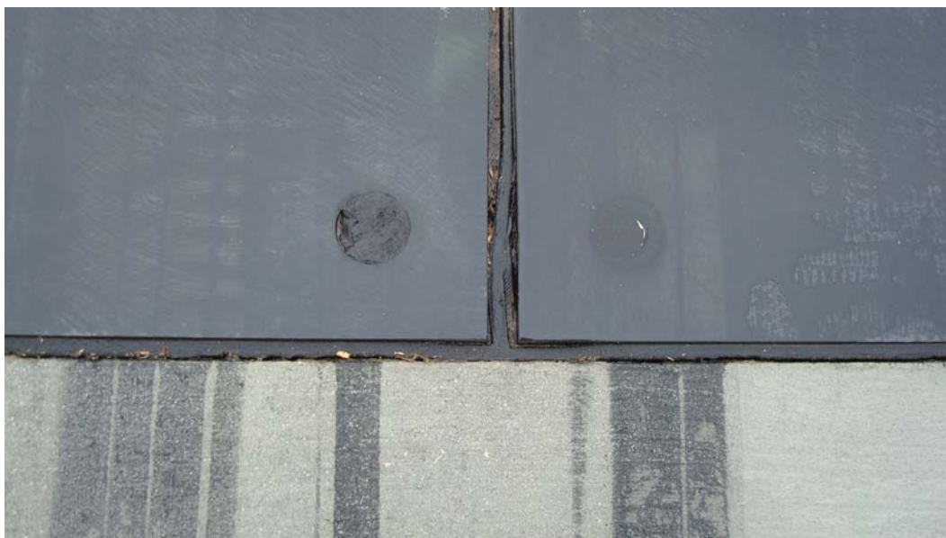
Figure 76. Performance of joint sealants at Runway 4 L at Shaw AFB.
