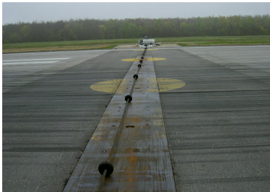
Figure 3. Use of steel plate at a Naval Base to protect pavement damage from cable.
