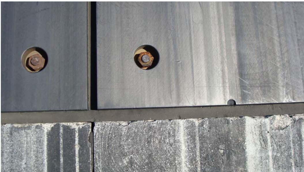
Figure 7. Sealant in good shape adjacent to panels at Aviano AB. Note lack of sealant in anchor bolt recess.
