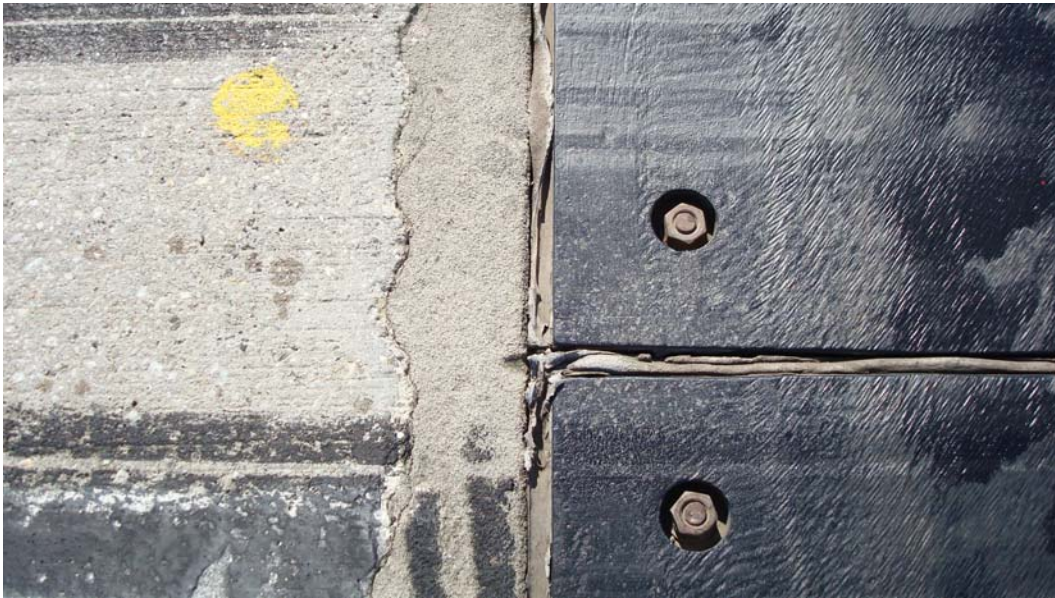
Figure 81. Repair of concrete adjacent to panels at Spangdahlem AFB.
