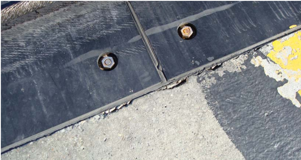
Figure 23. Typical spalling in concrete adjacent to panels at north end of runway at Eielson AFB.
