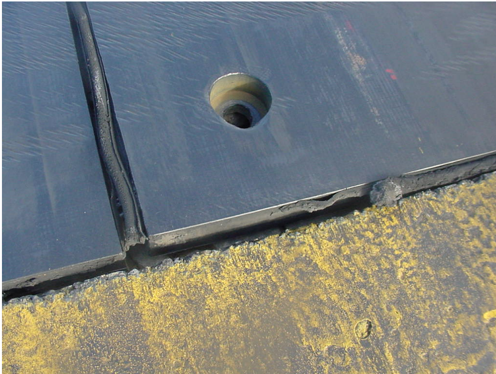
Figure 61. Loss of anchor bolt and nut at McChord AFB.
