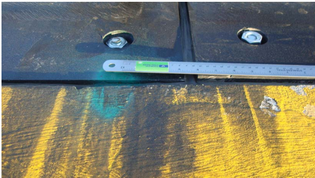
Figure 98. Some deviation in elevation of panels at Runway 13 R at Tyndall AFB.
