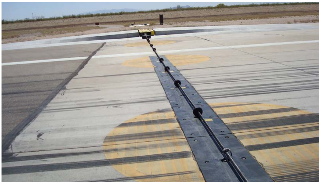
Figure 14. UHMW polyethylene panels at Davis-Monthan AFB within approximately 10 ft of change in pavement type.
