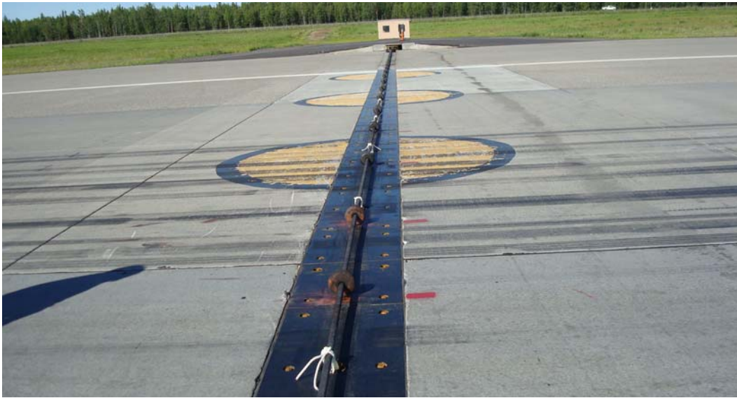
Figure 19. Overview of UHMW polyethylene panels at Eielson AFB showing concrete on both sides of the panels (south end of runway).
