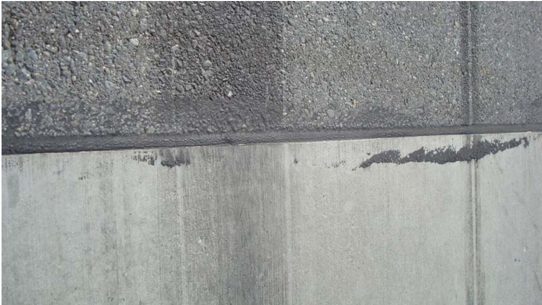
Figure 35. Condition of sealant between the concrete and asphalt pavements was generally good on Runway 24 at Elmendorf AFB.
