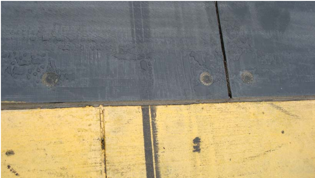
Figure 73. Performance of sealant and offset of joints in panels and concrete on Runway 22 L at Shaw AFB.
