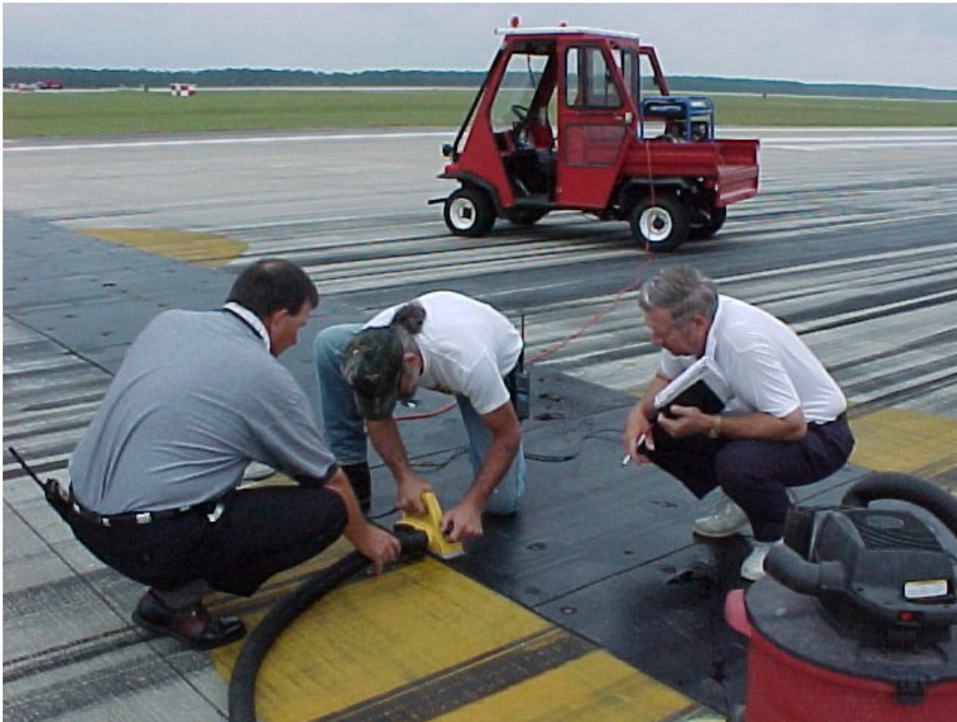
Figure 104. Grinding surface of panel to make smooth.
