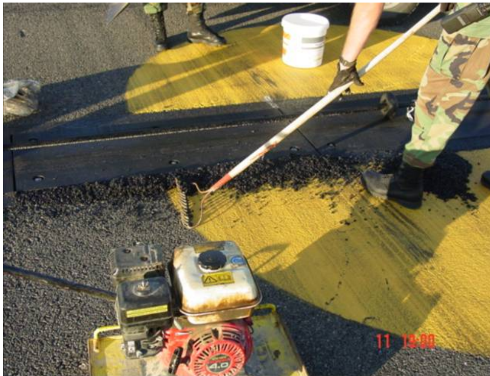
Figure 102. Fill hole with mix, level, and compact.
