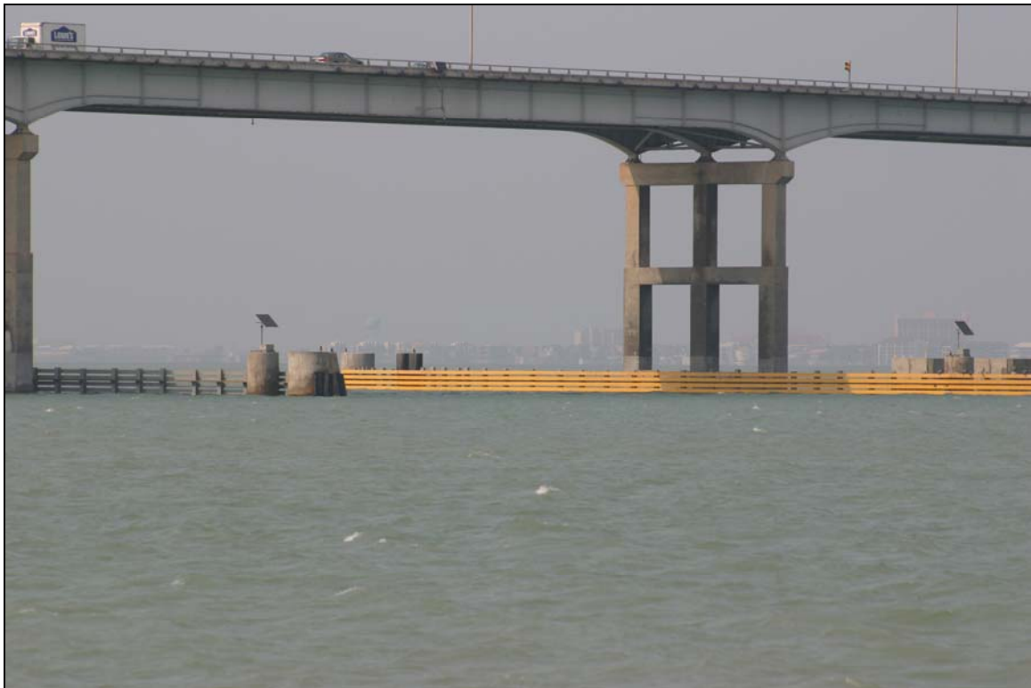
Figure 4. Queen Isabella Causeway and fender system.
