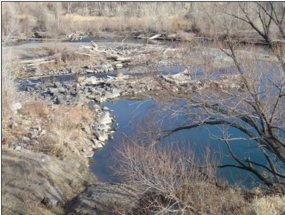
Figure 2. Large woody debris (LWD) removed from the stream bed and placed on the bank and mid-channel bar as a woody revetment to restore flow in the stream.
