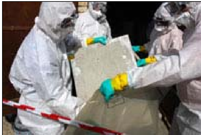
Figure 13. Safe handling of asbestos debris during disaster recovery requires respiratory protection and protective clothing. This protective equipment can stress relief workers, especially since most severe storms occur during hot times of the year.
