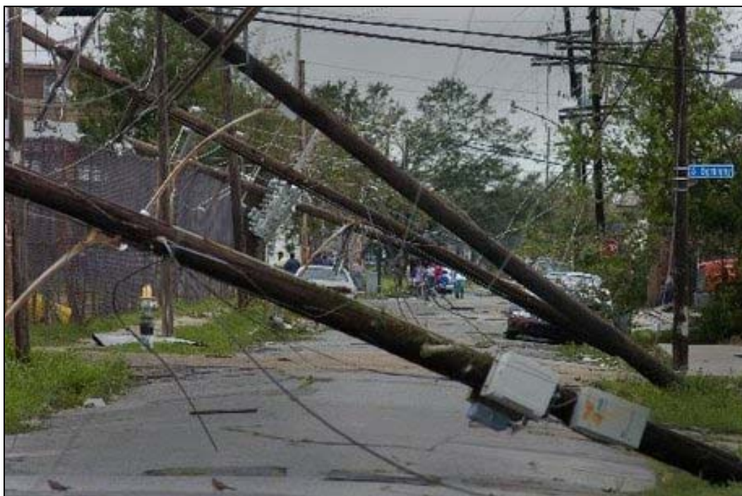
Figure 9. Fallen telephone poles resulting from Hurricane Katrina. These damaged poles are a source of CCA-treated wood. Photo provided by USACE.
