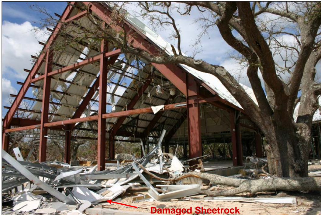
Figure 8. Damaged church near the Mississippi Coast following Hurricane Katrina. Damaged sheetrock is visible in the foreground. Photo provided by the MS-ASCE.
