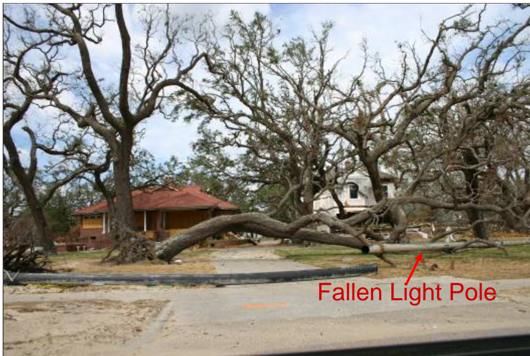
Figure 4. A fallen tree on the Mississippi Coast following Hurricane Katrina. The tree knocked down a light pole (see bottom right). Photo provided by the Mississippi Section of the American Society of Civil Engineers. MS-ASCE.
