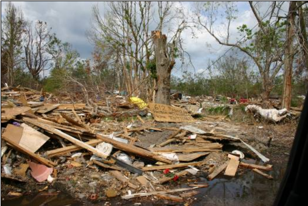
Figure 5. Completely destroyed homes near the Mississippi Coast following Hurricane Katrina. Photo provided by the MS-ASCE.
