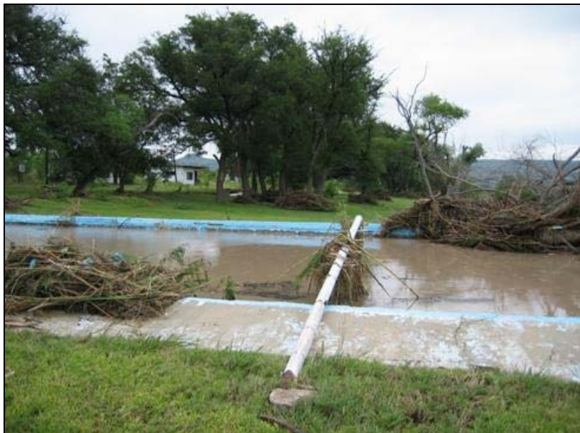
Figure 18. Swimming pools filled with debris can rapidly become health hazards to the community. This is a pool in Southern Mississippi following Hurricane Katrina. Photo provided by USACE.
