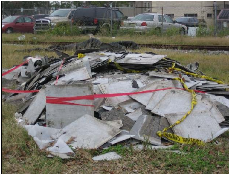
Figure 12. Removed asbestos-containing material resulting from Hurricane Katrina. Material was marked so it would not be picked up by hauling crews. Photo provided by USACE.
