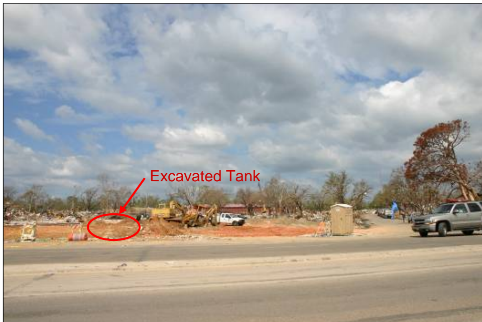
Figure 11. An exposed, excavated underground storage tank near the Mississippi Coast after Hurricane Katrina, illustrating the potential for chemical release. Photo provided by the MS-ASCE.
