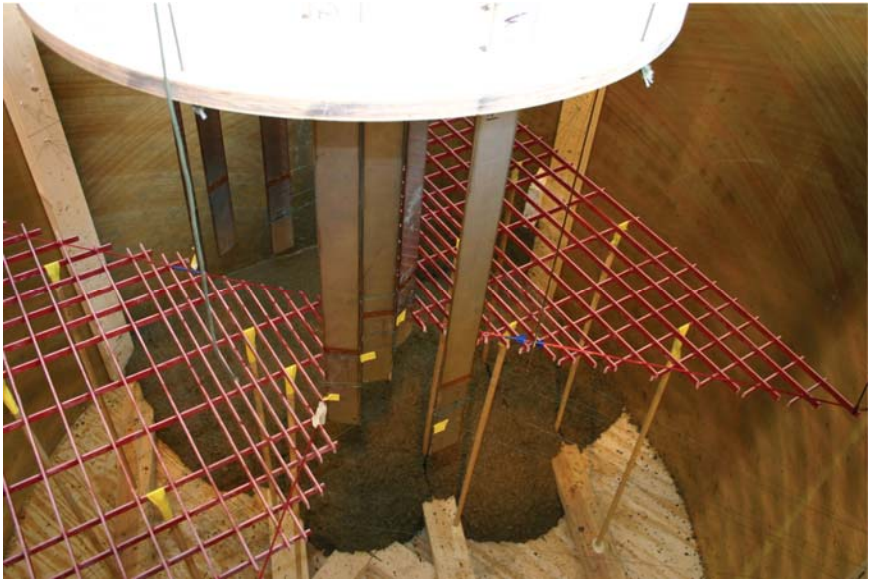
b. Concrete placement.
