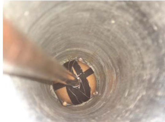
b. Charge in precast hole.
