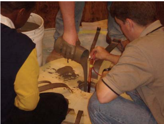
c. Grout backfill.
