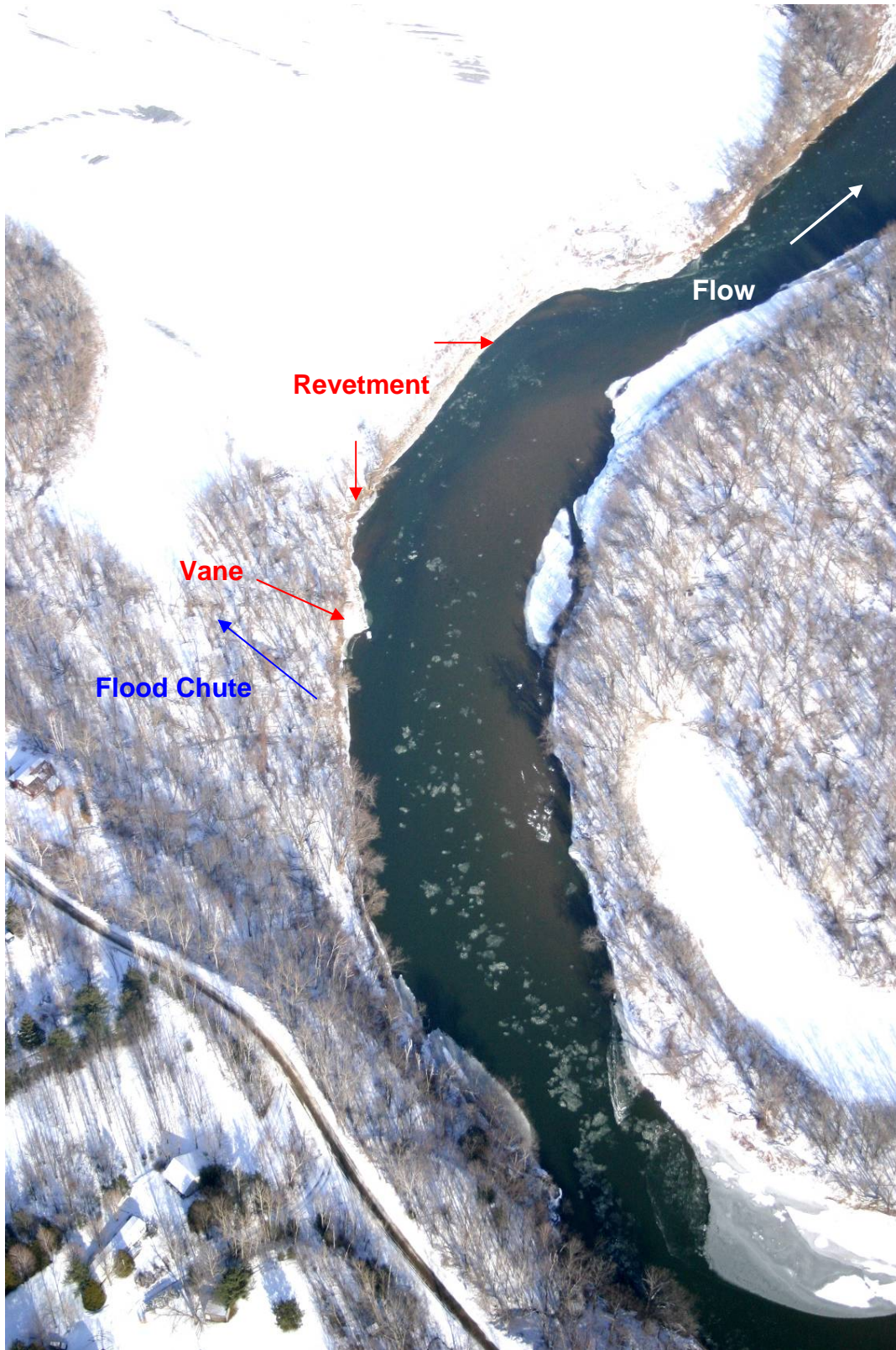
Figure 16. Frazil pans drifting past vane and revetment at the Snowflake Farm property downstream of Richmond, VT, 1/31/08.
