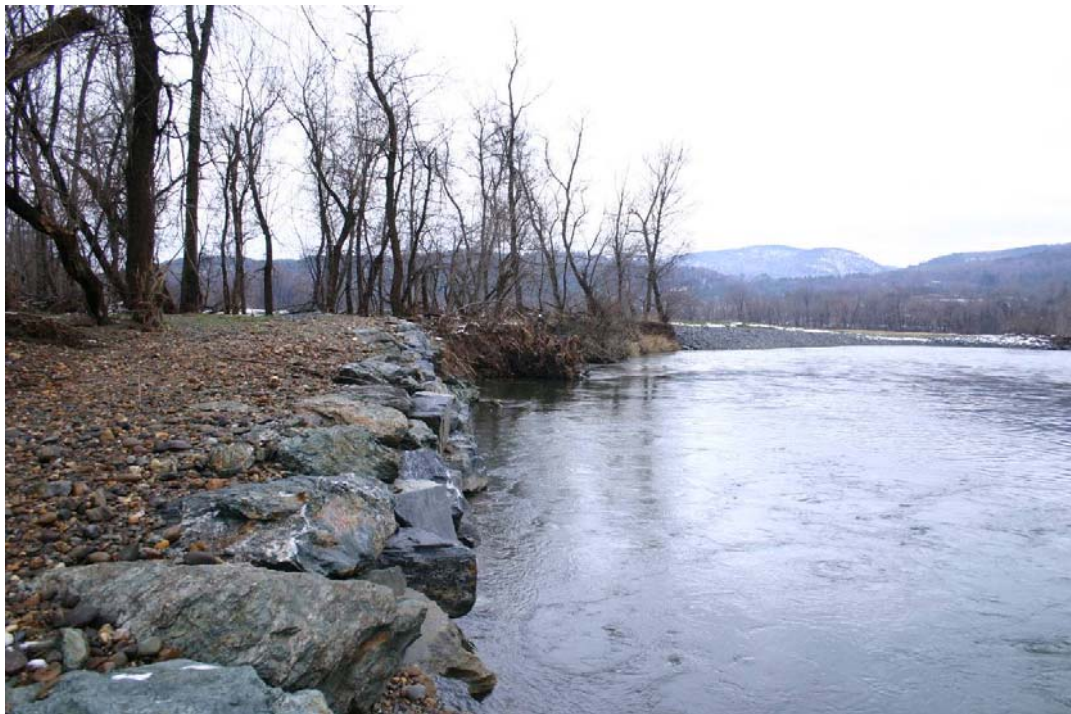
Figure 17. Vane and revetment at Snowflake Farm viewed from upstream on 11/28/05.
