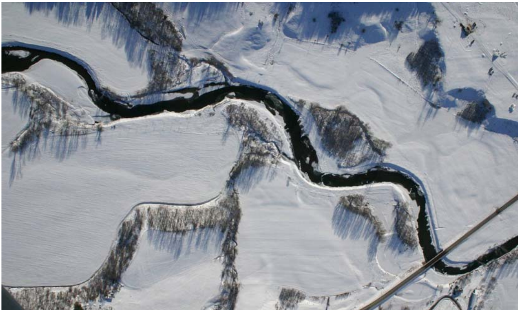
Figure 38. Trout River looking at the East Berkshire Bridge restoration project on 1/4/06.
