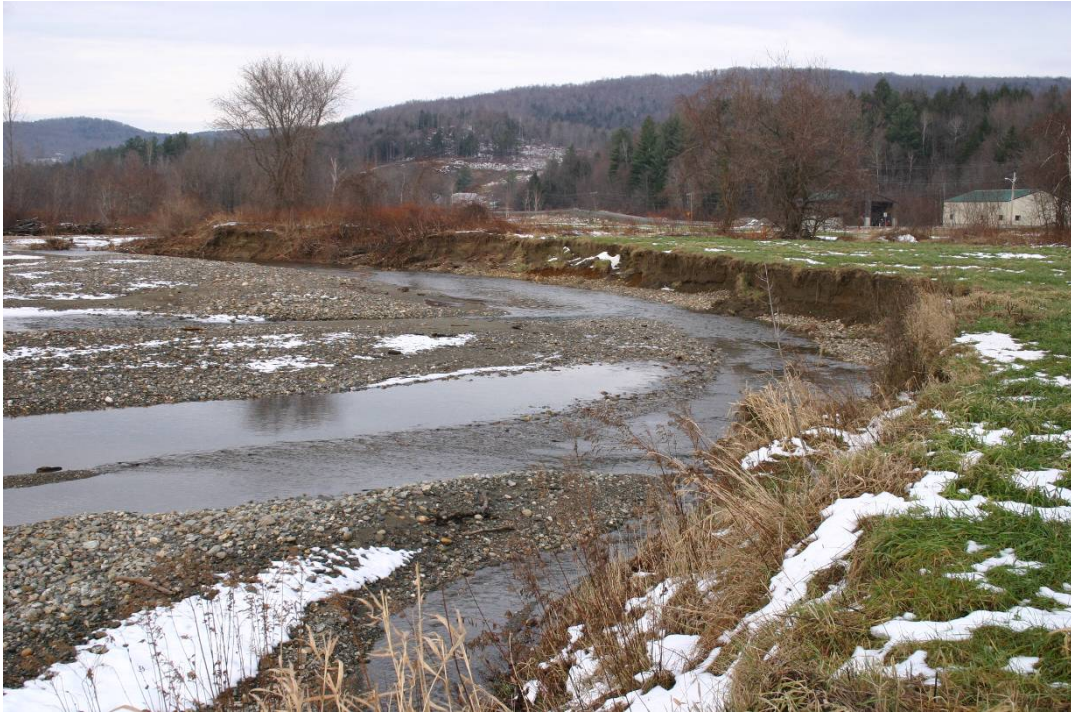
Figure 33. Trout River looking downstream at eroding bank on 11/28/09.
