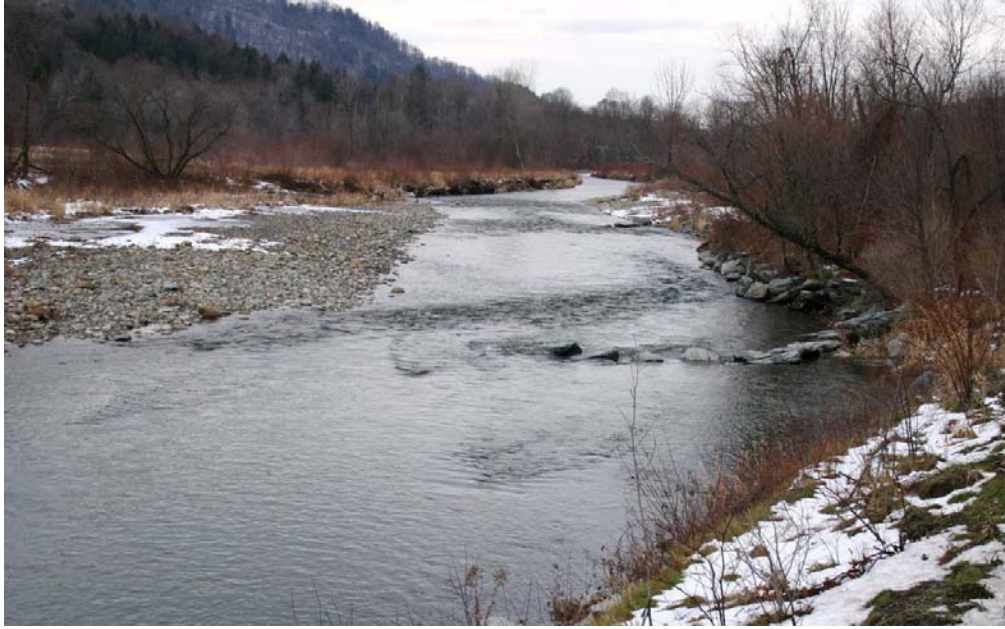
Figure 30. Cross vanes stabilize banks of channel diverging from Rt. 118 on the Trout River 11/28/05
