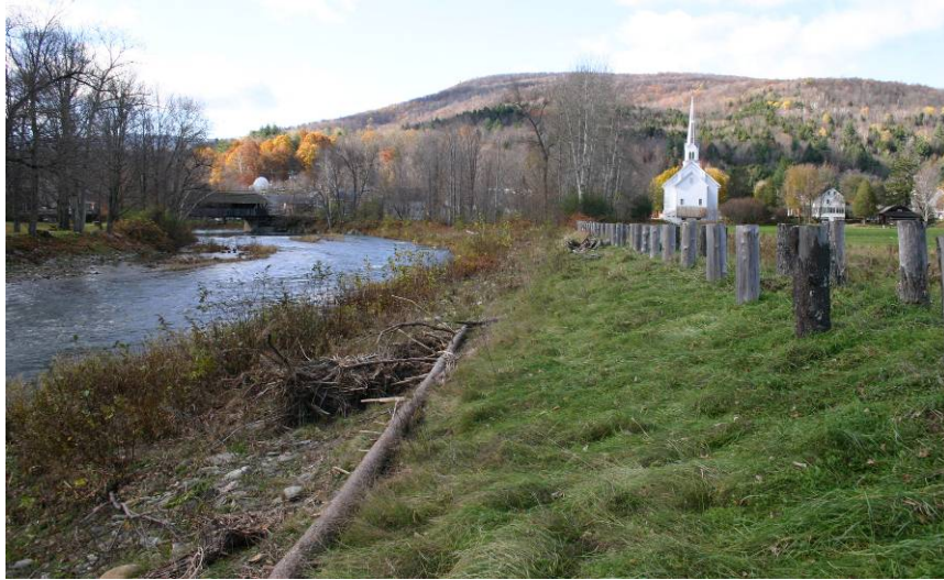
Figure 26. Mad River at Waitsfield: Ice retention posts 11/2/05.
