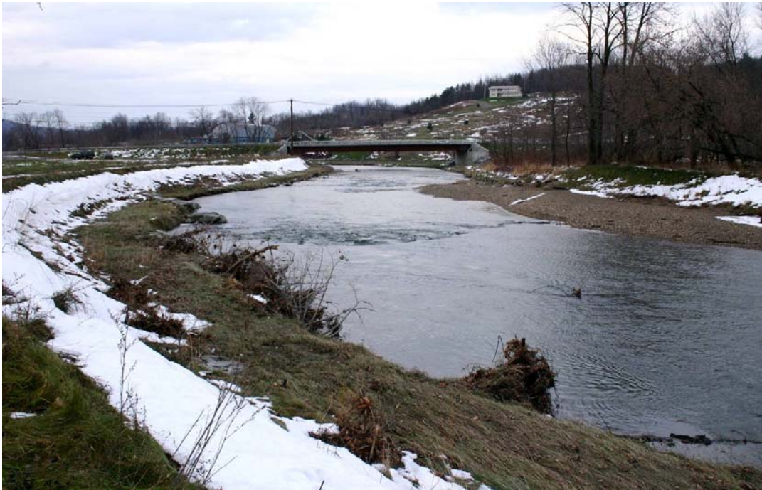
Figure 36. Trout River looking downstream at a U-drop and rock riffles at the East Berkshire Bridge restoration project on 11/28/05.
