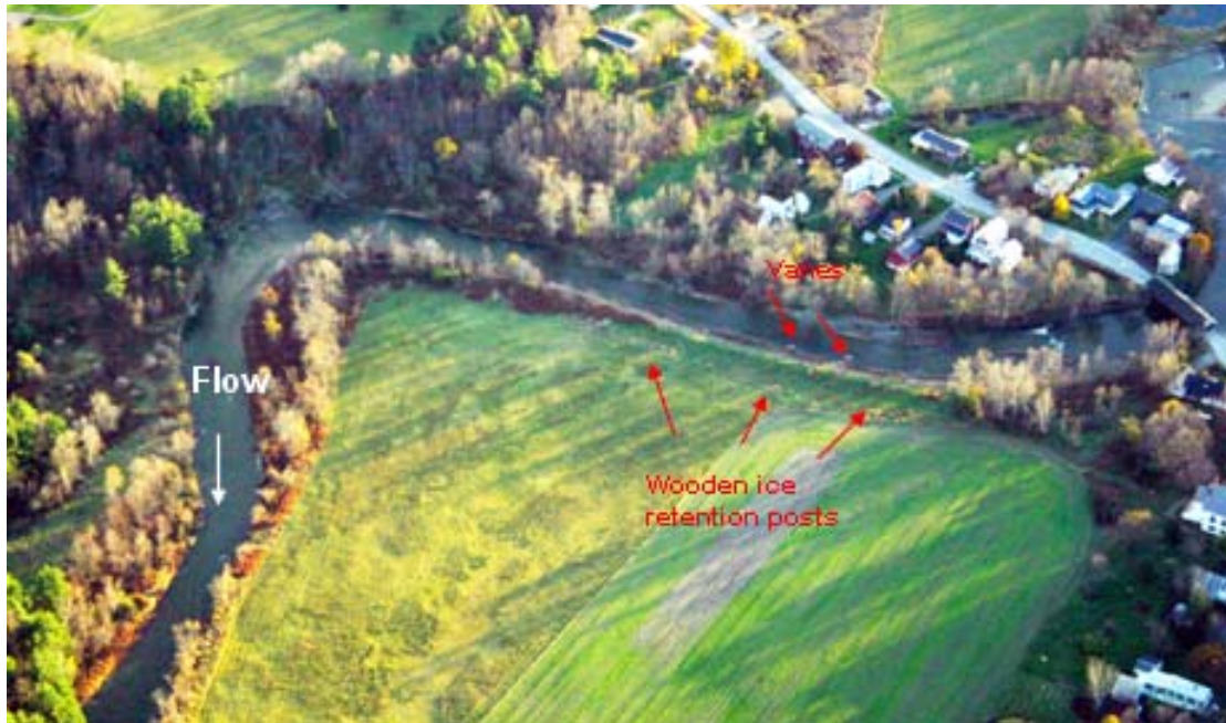
Figure 25. Mad River at Waitsfield: Site of two small rock vanes and ice retention posts. 11/2/05.
