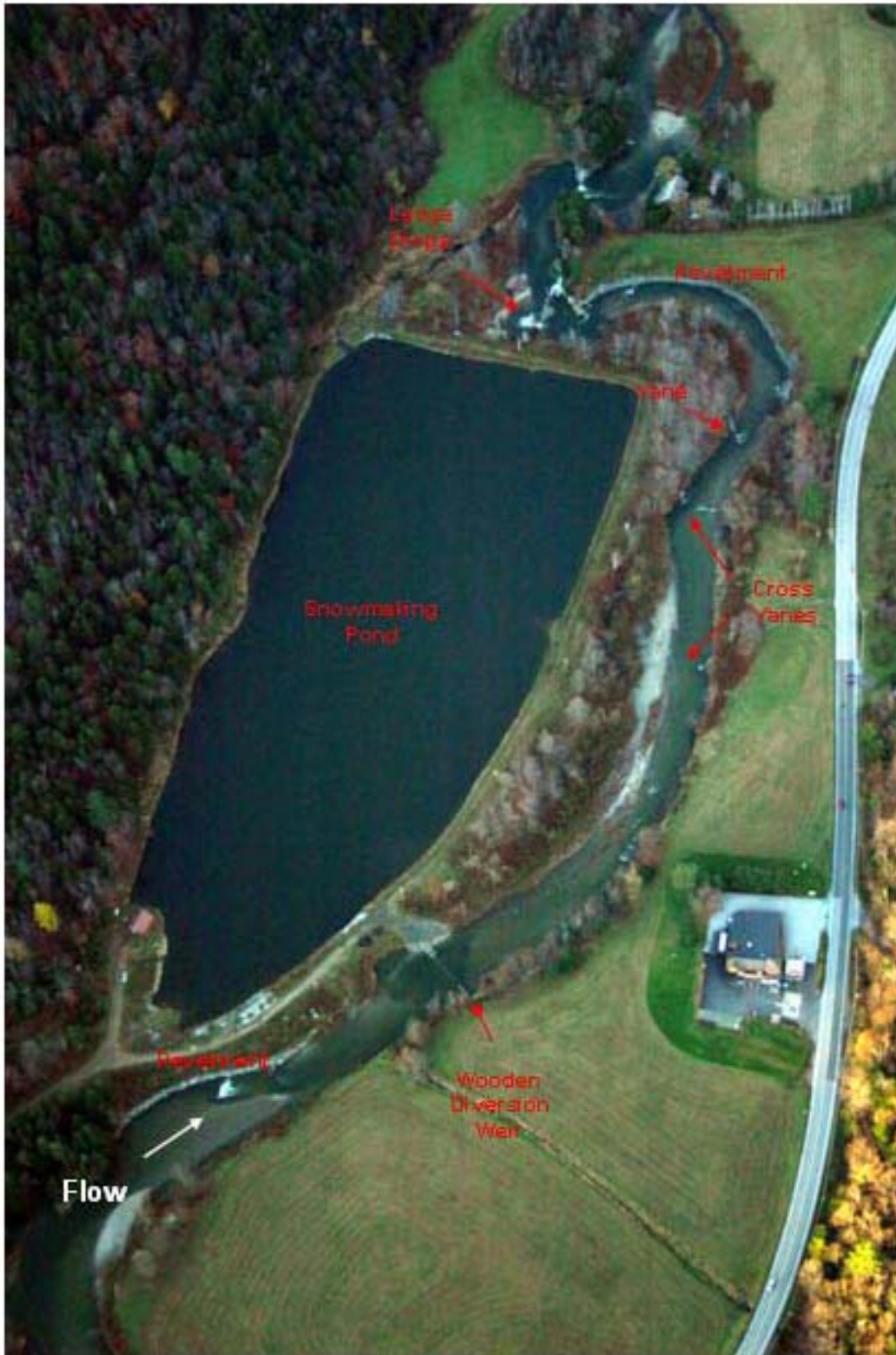
Figure 22. Channel restoration structures on the upper Mad River at the Warren snowmaking ponds. 11/2/05
