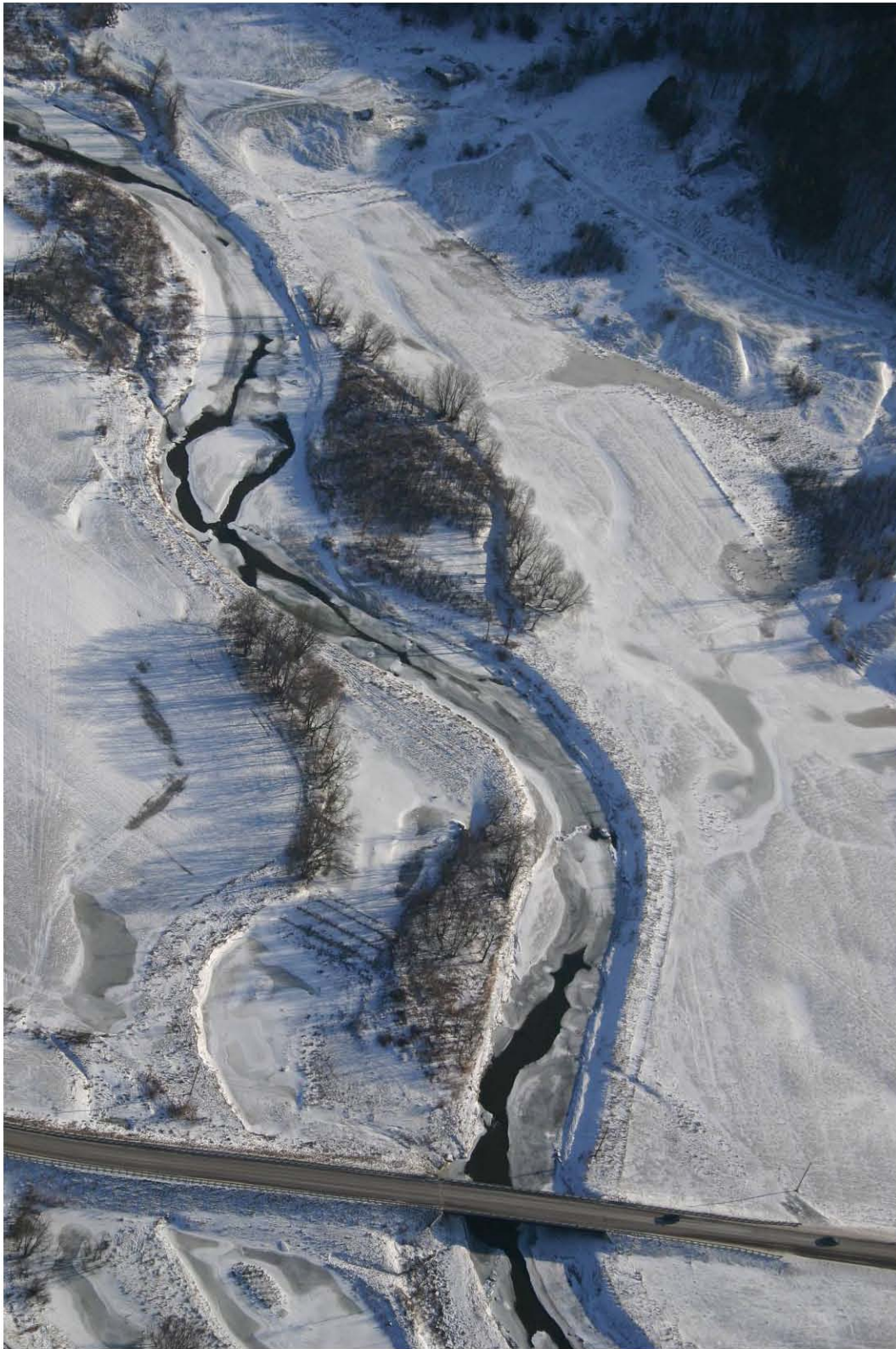
Figure 39. Trout River East Berkshire Bridge restoration project on 1/31/08.
