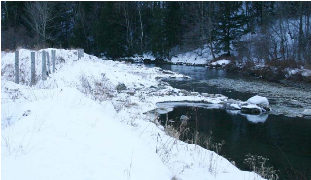
Figure 41. Vanes stabilizing bank of the White River above Rochester, VT. 1/10/06. Posts and berm to prevent ice from escaping into field of left.
