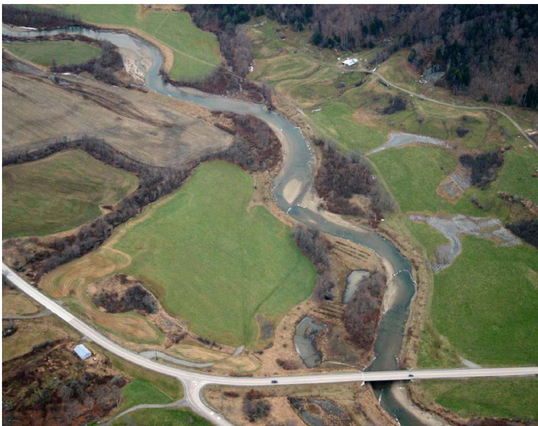
Figure 37. Trout River looking upstream at the East Berkshire Bridge restoration project on 12/3/08.
