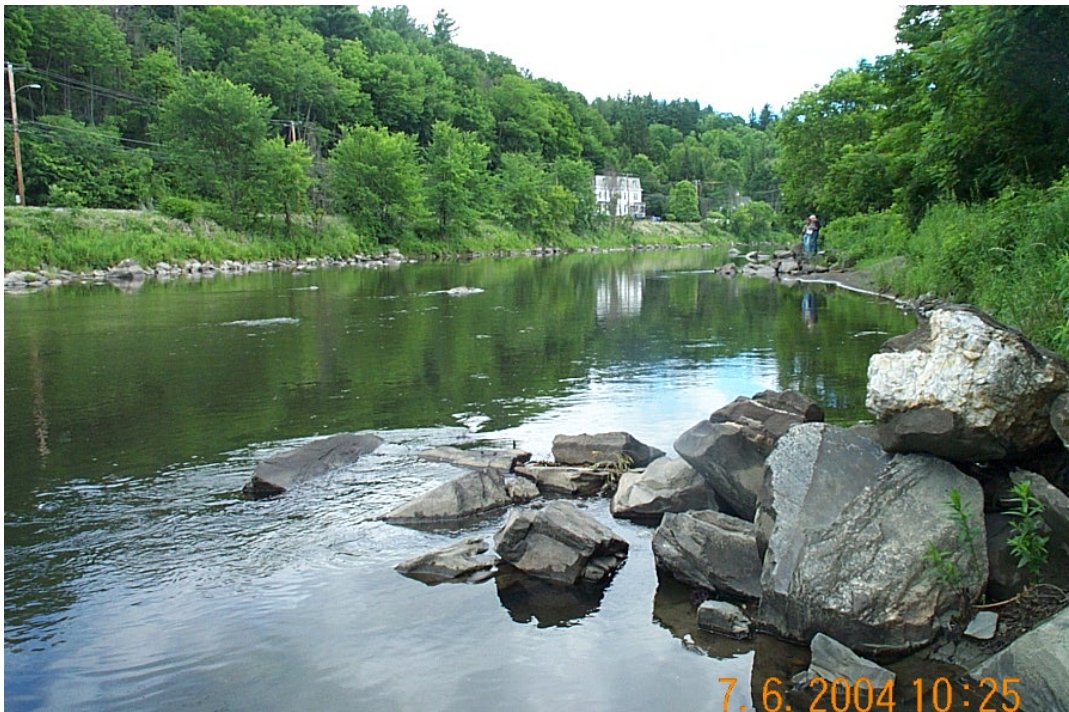
Figure 11. Rock vanes on the Winooski River at Montpelier, VT viewed from downstream on 7/6/04.
