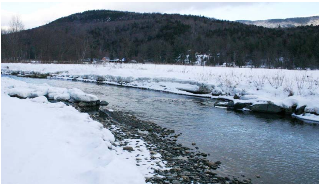
Figure 40. Cross vane stabilizing banks of the White River below Granville, VT following mid-winter breakup 1/10/06.
