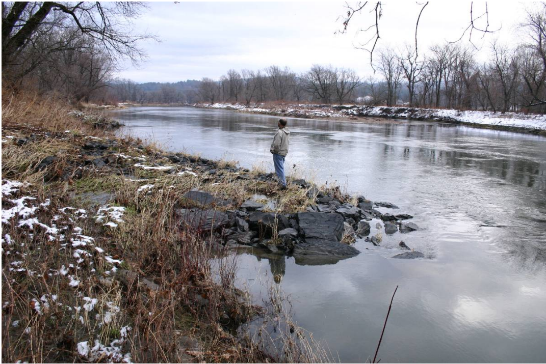
Figure 19. Cross vanes on the Winooski River along Gov. Chittenden Rd. viewed from upstream on 11/28/05
