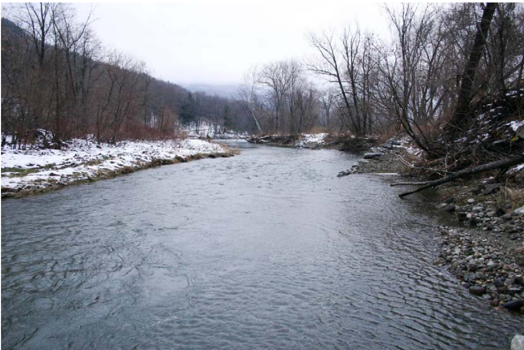
Figure 14. Rock vanes on the Winooski River, Fuller Farm, Bolton, VT viewed from upstream on 11/2/05.
