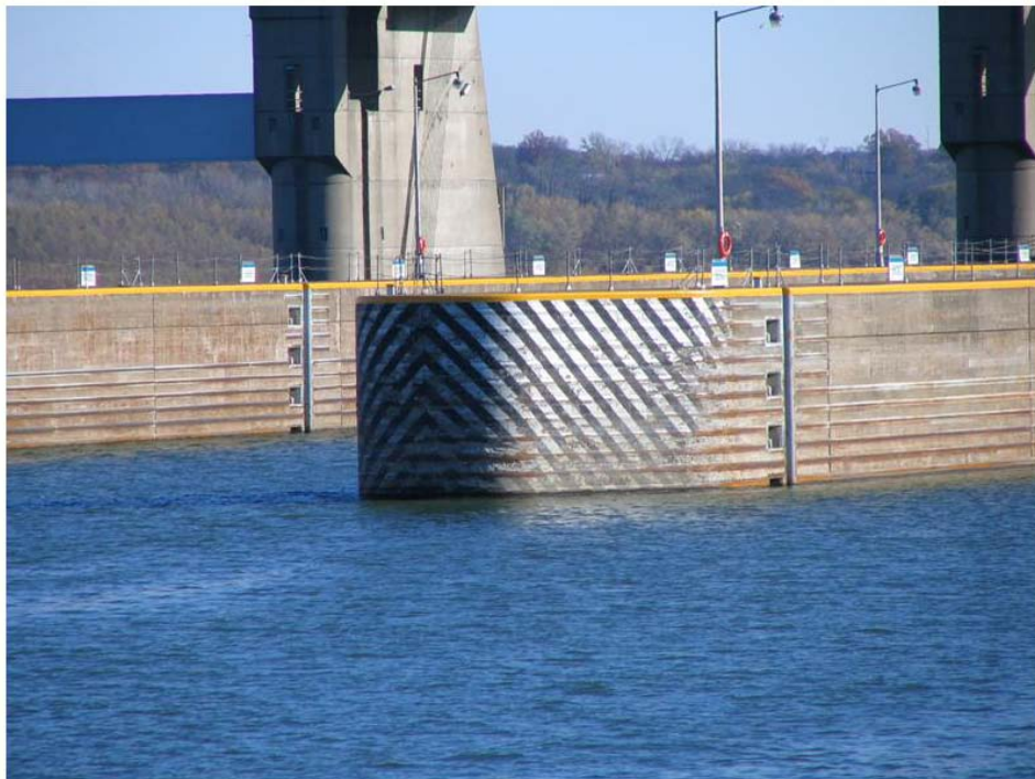
b. Closer view of the bullnose, upper middle wall.
