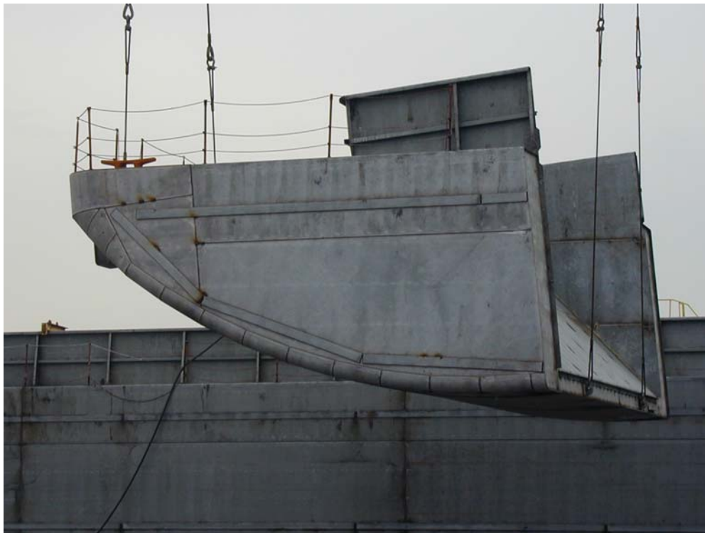
Figure 2.1. Side view of the bow of a raked section, jumbo open-hopper barge.
