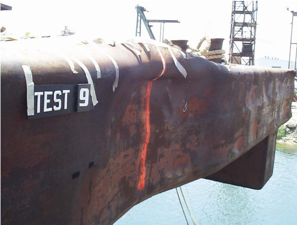
Figure 3.21. Crushing damage of barge headlog (from HQUSACE 2004).
