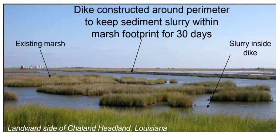
Figure 7. Dike constructed on backside of island at Chaland Headland to retain fine clay, silt, and mud during marsh construction
