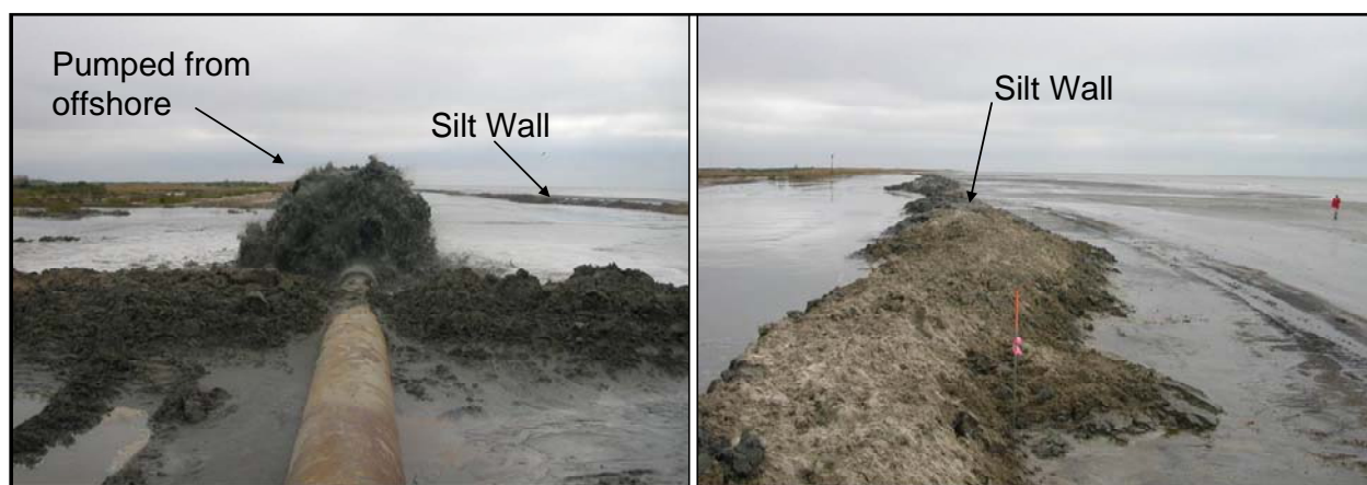
Figure 6. Dike constructed on Gulf beach at Chaland Headland, LA, to retain fine sand and silt during placement.
