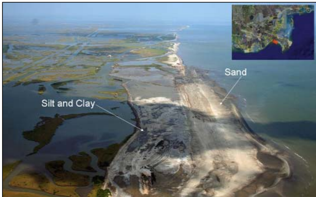
Figure 6. Chaland Headland, Louisiana restoration project during construction showing different types of sediment placed (looking southeast, 1 September 2006).
