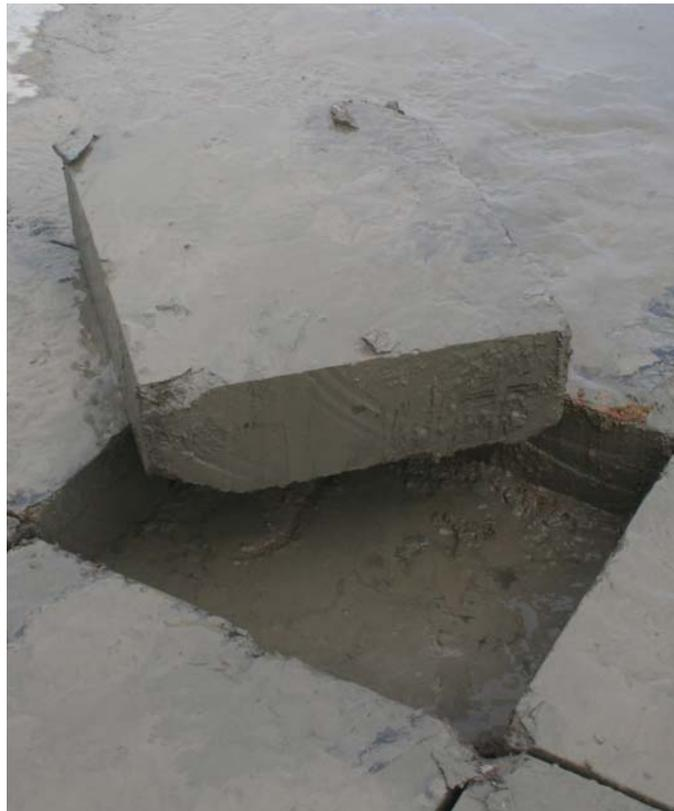
Figure 12. Recovered stabilized surface slab sample.
