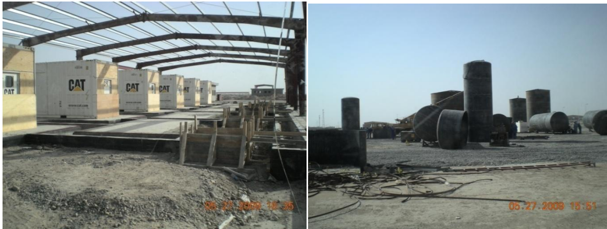
Figure 5—Diesel Generators and Fuel Tanks
