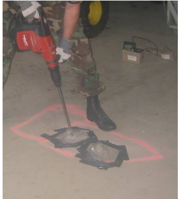
Figure 6-3. Example of Fixed Contamination Removal by Rotary Hammer (Shelter 210).
