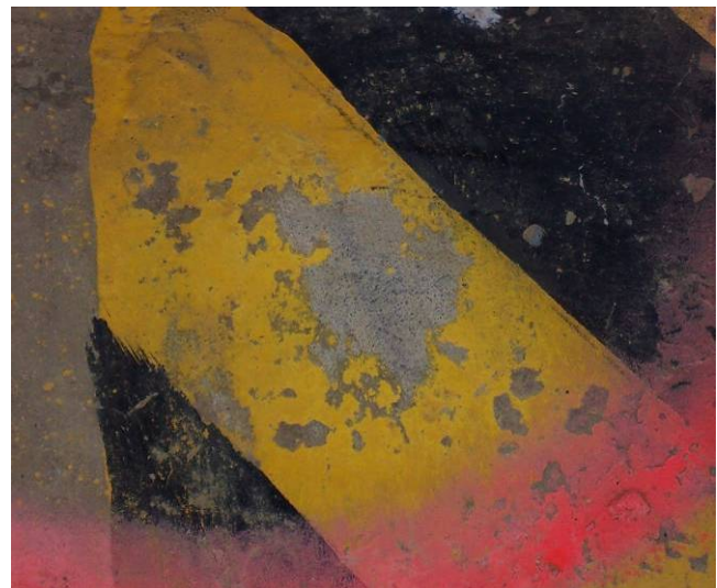
b. Post Abrasive Removal.
