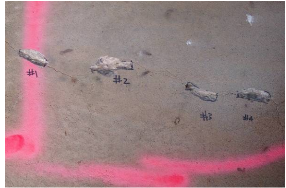
b. Areas Following Hand Chisel Mitigation
