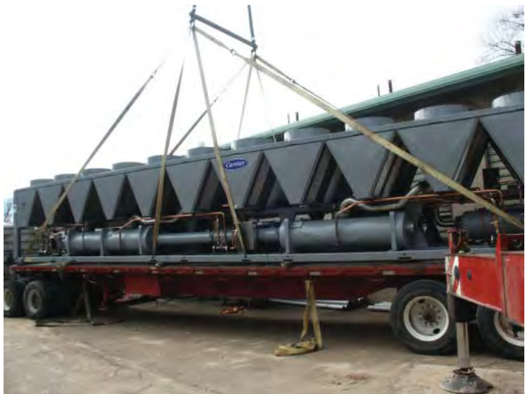
Figure 2. Delivery of 500 ton chiller
