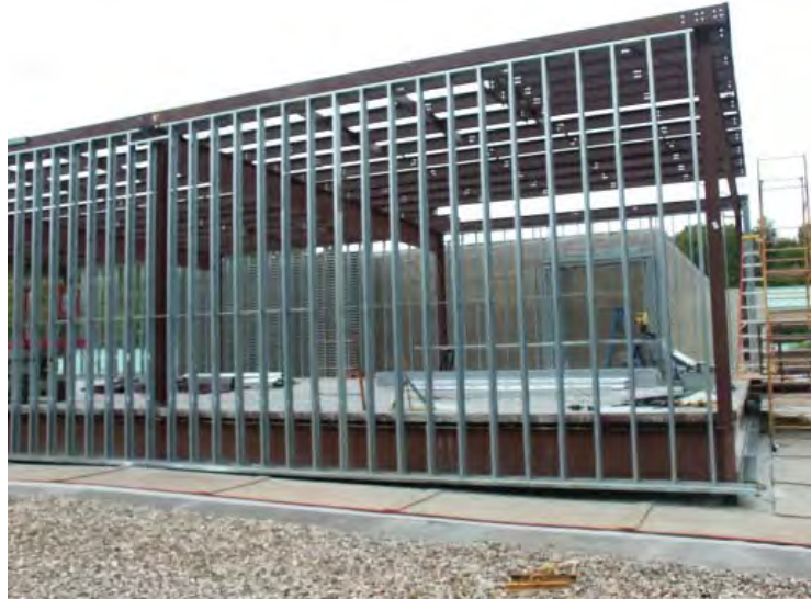
Figure 1. New UPS equipment shelter located on the roof of ERDC Information Technology Laboratory building
