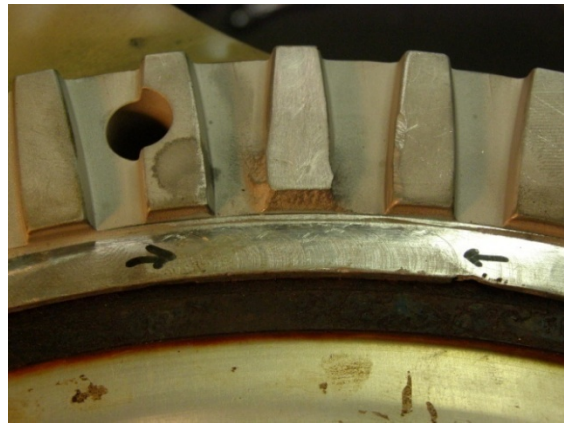
Figure 30. Cold spray aluminum fill machined back to the original dimensions.
