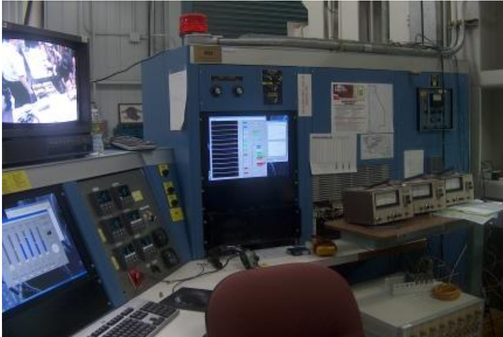
Photograph #5: Instrumentation Station for Manned Testing
