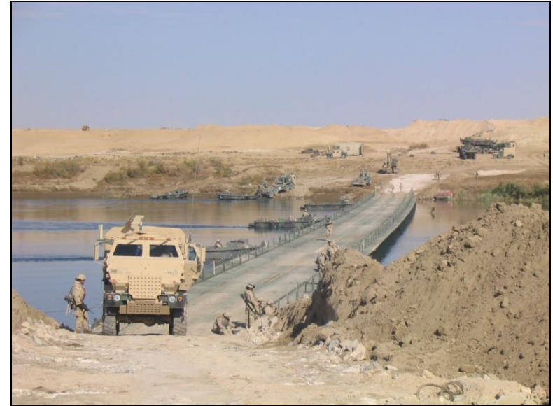
Standard Ribbon Bridge bays in Bridge configuration Bridge Erection Boats provide temporary anchorage
