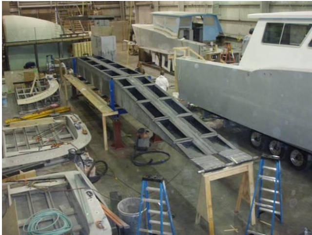
Internal view of Treadway without Deck
