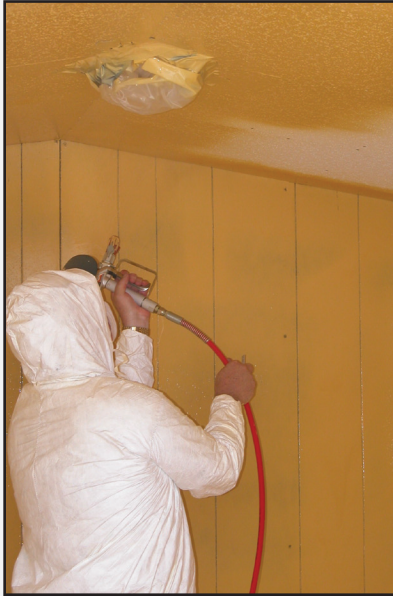
AFRL research scientist Mr. Scott MacLean applies a barrier coating to a large-scale test facility at Tyndall Air Force Base, Florida.
