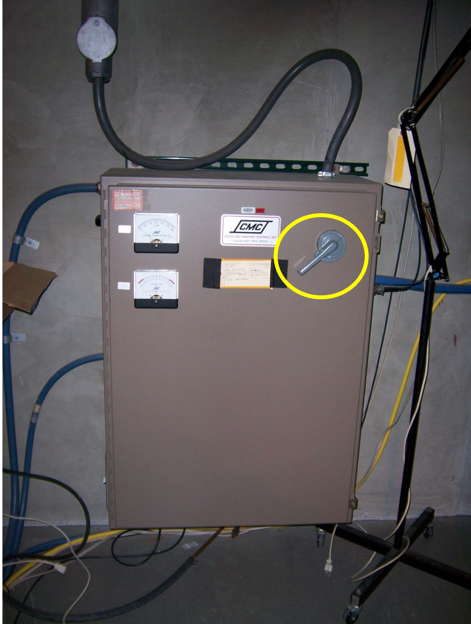
Figure A.8. Centrifuge table motor control power switch.
