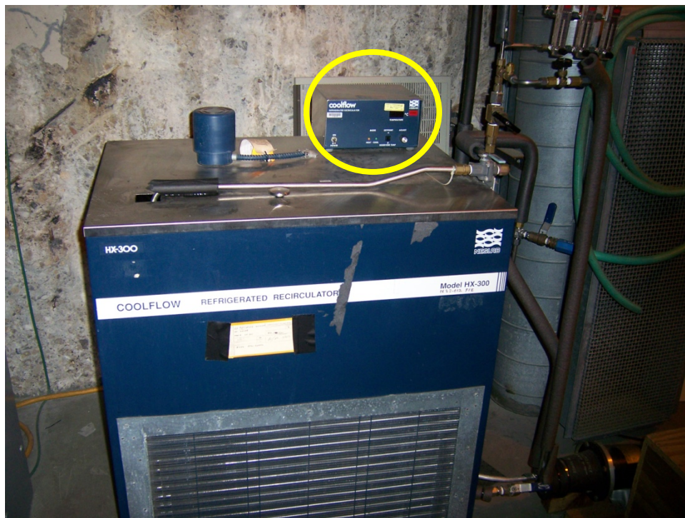
Figure A.5. Neslab recirculating chiller.
