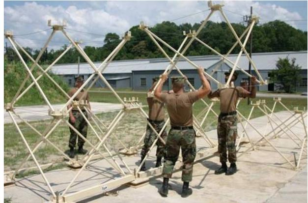
Figure 2 Linking and stacking MPS frames
