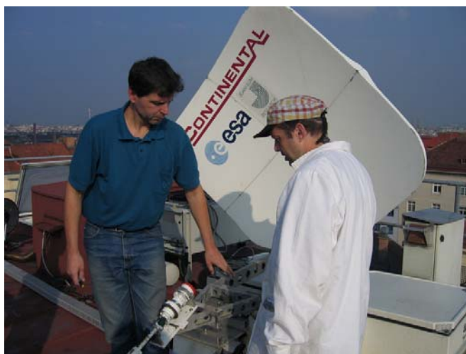
Figure 1. Bernd Blanzano and Werner Mache during installation of the TUG03 antenna on top of the BEV building.
