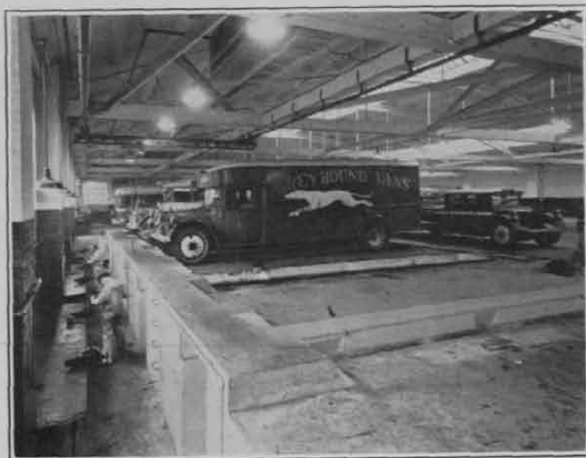
Plate 5. Maintenance Pit Showing Connection with Header Pit. Note overhead Crane Trolley for Removal of Heavy Parts.
