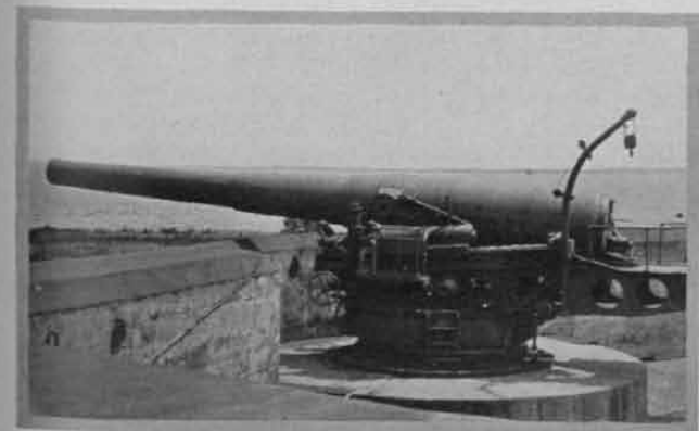
Figure 1. Showing Number 1 gun, 12-in B. C., before base ring leveling operation was commenced.
