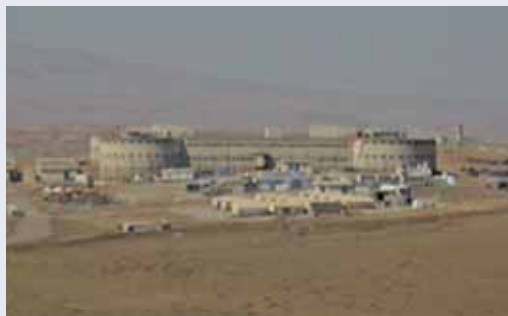
Construction was 63% complete this quarter at Fort Suse Prison in Sulaymaniyah. (USACE photo)
