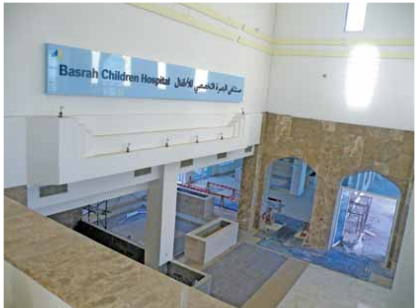
Entry corridor in the main hospital building of the Basrah Children’s Hospital.
