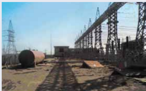
Substation Najaf project is almost complete. (USACE photo)
