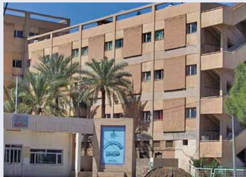
The concrete shell is almost complete for the surgical wing of Ba'quba General Hospital in Diyala province. (USACE photo)
