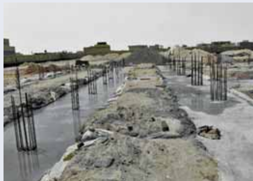
Steel columns protrude from the foundation of the Al Semood Secondary School in Kerbala. (USACE photo)
