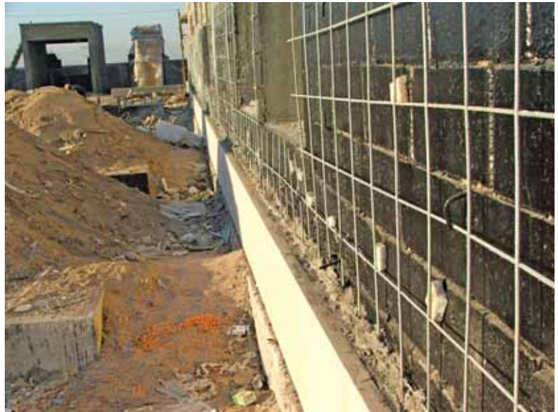
Exterior stone cladding installation at the Basrah Children's Hospital.
