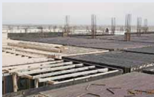
The foundation is laid for the surgical hospital in Missan. (USACE photo)
