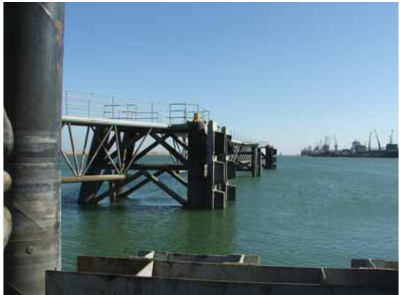
SIGIR's inspection of the $2.7 million IRRF-funded Roll-On/Roll-Off Berth in the Port of Umm Qasr found only minor construction deficiencies.
