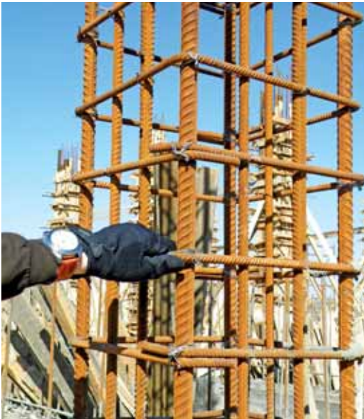
Example of constructed column section at the Missan Surgical Hospital.
