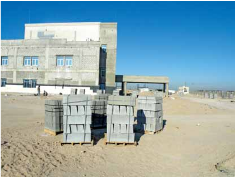
Curb stones and grading work for parking at the Basrah Children's Hospital.
