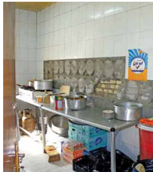
Damaged kitchen wall and tiles in the 4th Brigade 10th Infantry Division kitchen.
