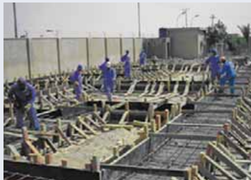
Workers lay the foundation of the Water Reverse Feeding Project in Garma, Basrah province. (USACE photo)
