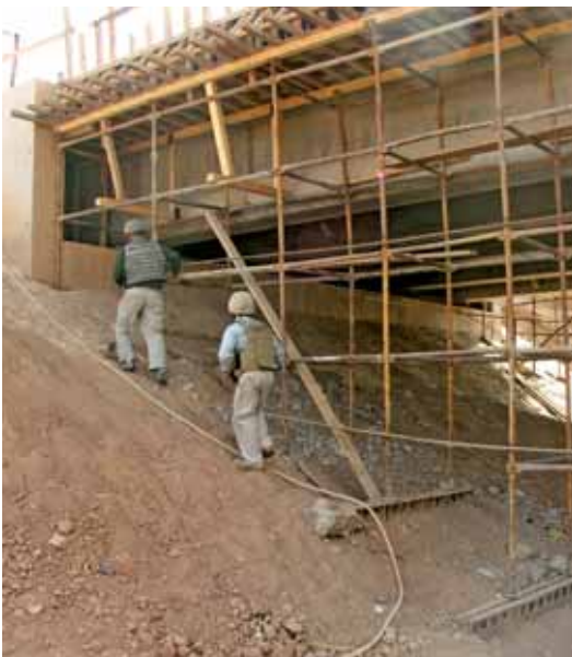
Inspectors at the Mujarrah Canal Bridge.
