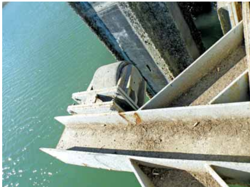
Cushion rollers with steel spacer plates at RORO Berth.
