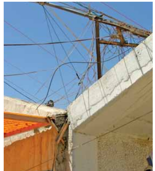
Electrical wiring connecting to system.
