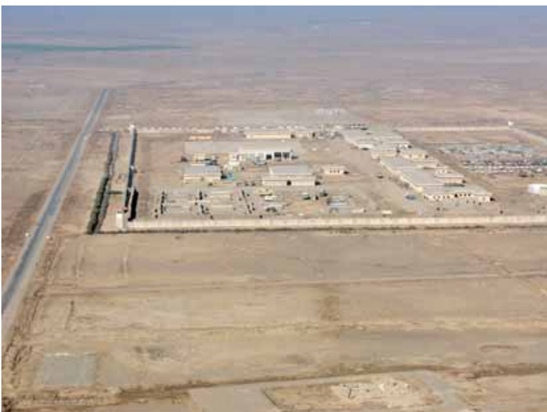
Overhead view on approach to the 4th Brigade 10th Infantry Division site.
