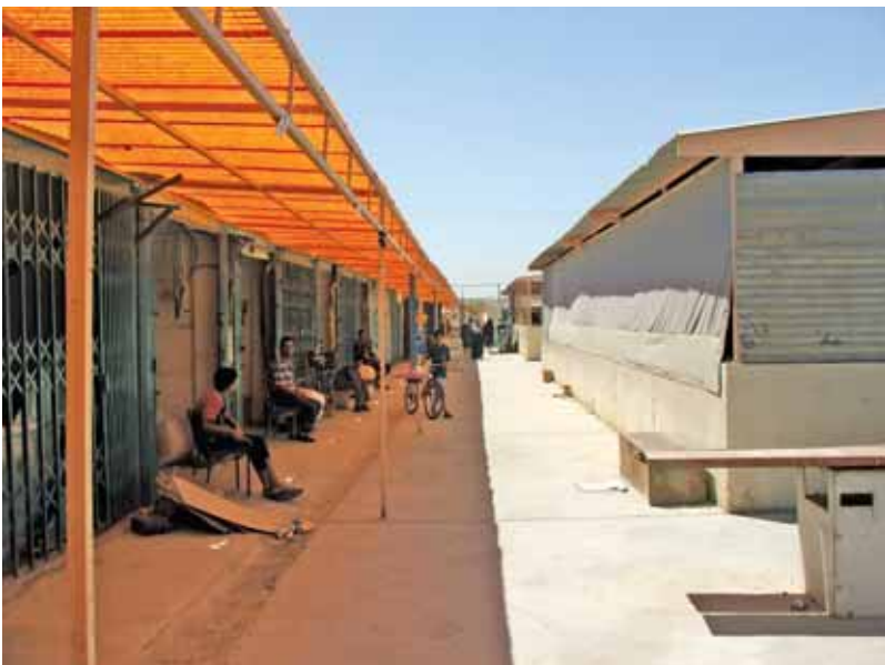
Slab along existing shops at the Ammana Market.
