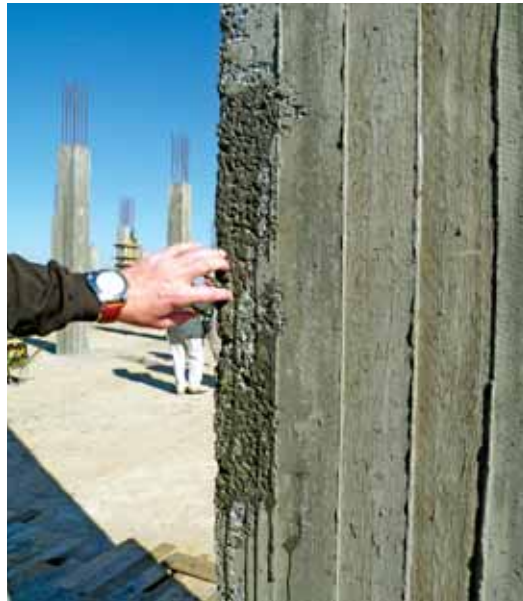
Example of concrete honeycombing in constructed columns at the Missan Surgical Hospital.
