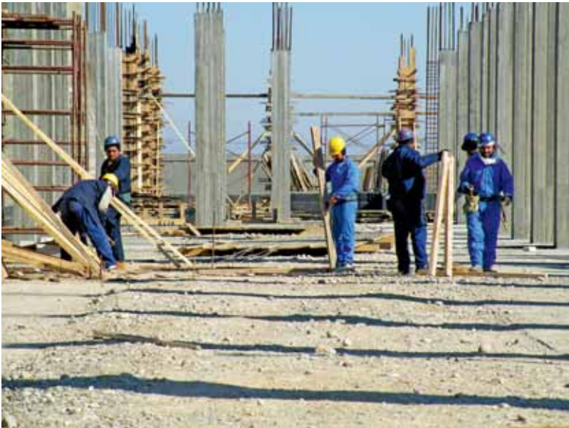
Ongoing construction at the Missan Surgical Hospital.
