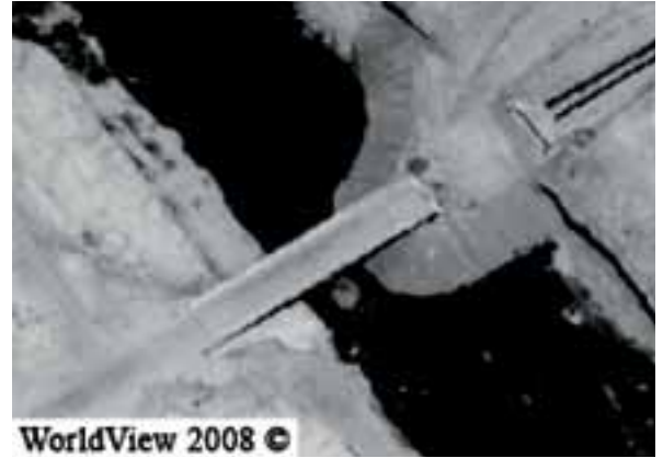
Imagery of the Mujarrah Canal Bridge (PA-09-170), taken on July 4, 2008.
