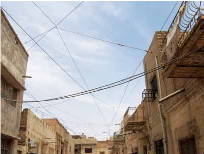
SIGIR's audit of the Muhalla 312 electricity expansion found that the contractor fulfilled project specifications.
