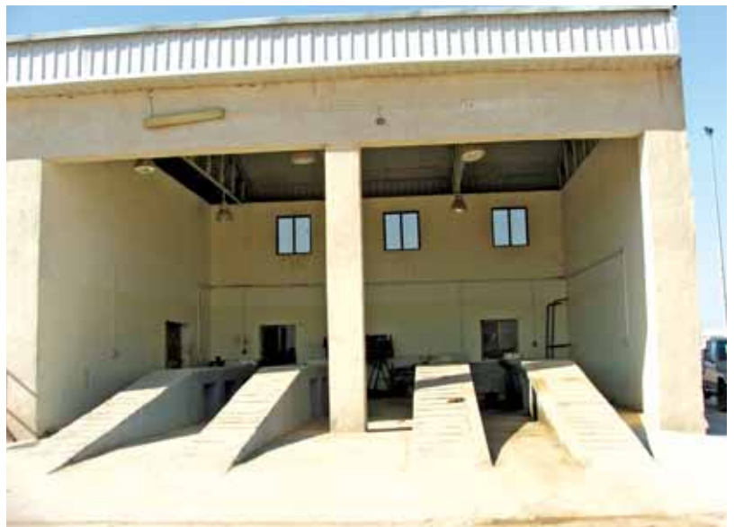
Equipment maintenance building at the 4th Brigade 10th Infantry Division facility.
