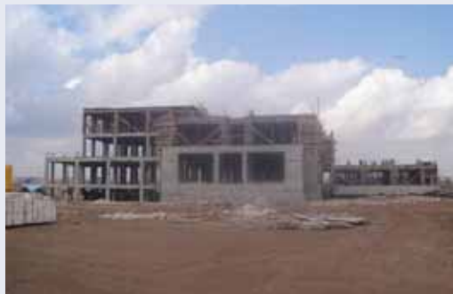
Skeleton of the Erbil Emergency Hospital. (USACE photo)
