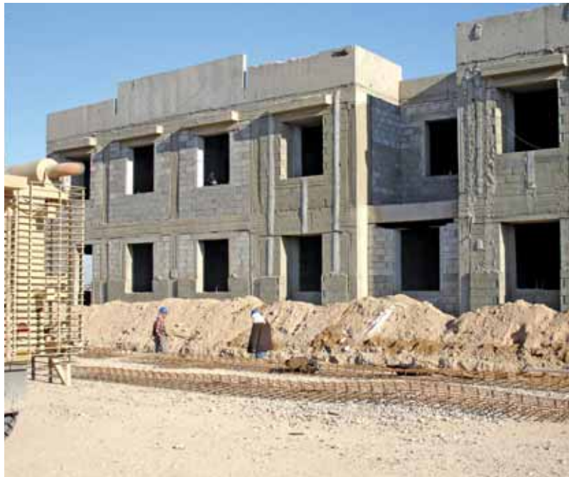
Ongoing construction work at the Basrah Children's Hospital.
