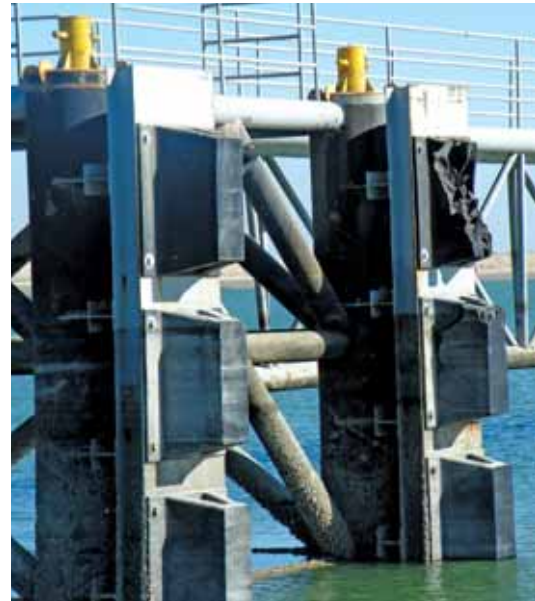
RORO Berth 22 sheared rubber fenders.
