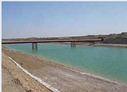
A new drain pipe crosses the Euphrates River in Muthanna. (USACE photo)
