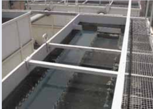
Construction of a new potable water filtration system in Al-Kasik, Ninewa. (USACE photo)
