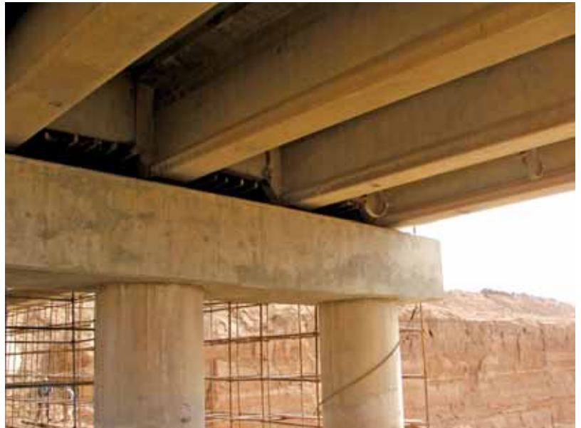
Bent cap at Pier No. 1 of the Mugarrah Canal Bridge.
