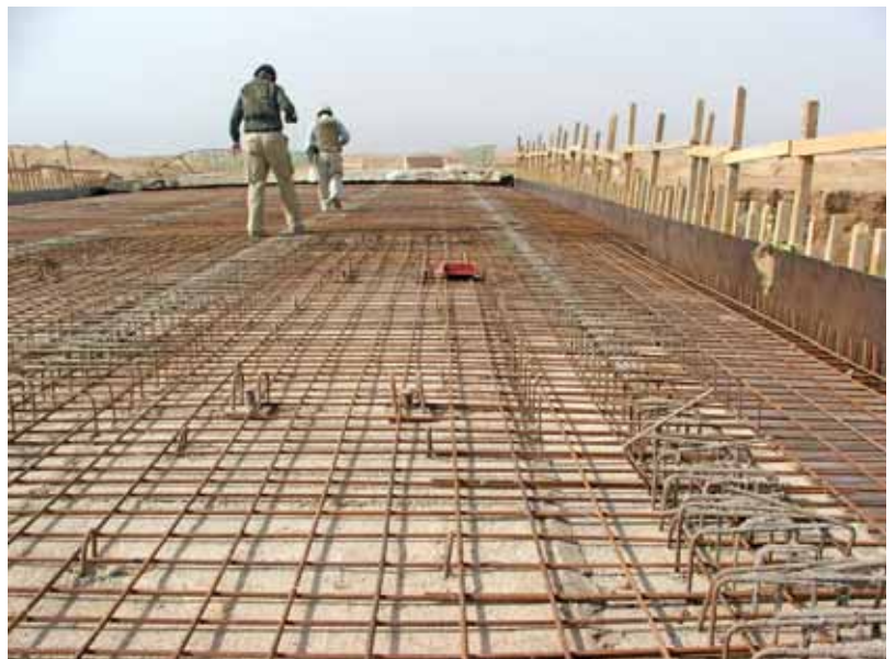
Concrete deck reinforcing (prior to placing top mat, foreground).
