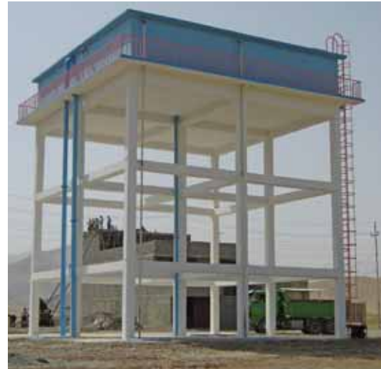
Workers construct the Rania Water Project in Sulaymaniyah province. (DoS photo)
