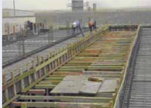
Workers lay the foundation for the Nassriya Prison. (USACE photo)
