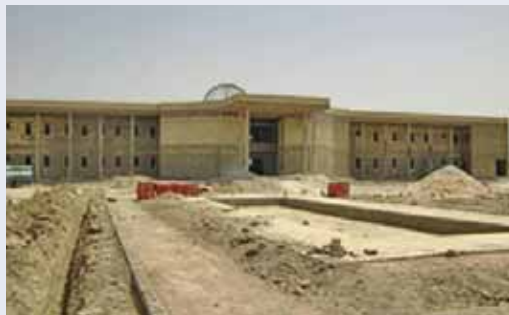
Concrete shell of the courthouse in New al-Hilla, Babylon province. (USACE photo)
