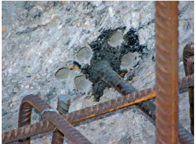
Foundation at Missan Surgical Hospital showing multiple holes surrounding epoxy-anchored dowel.
