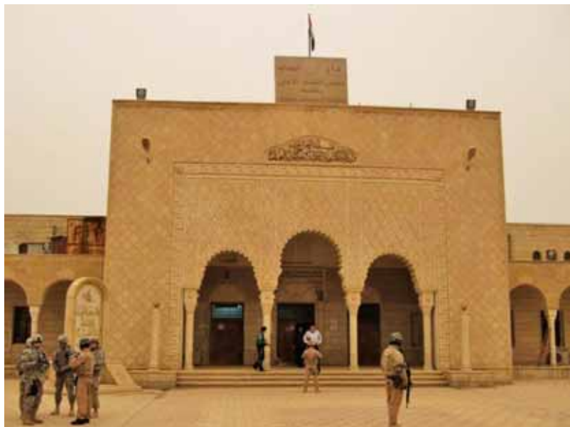
U.S.-funded renovation of the old Mosul Courthouse. (USACE photo)
