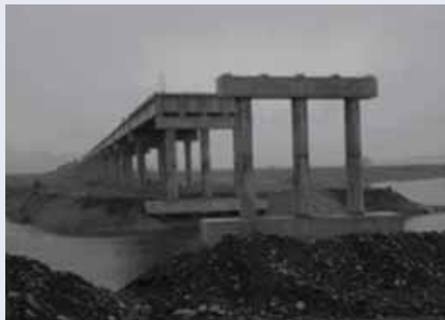
The first few pillars of the new al-Shirqat Bridge in Salah Al-Din. (USACE photo)
