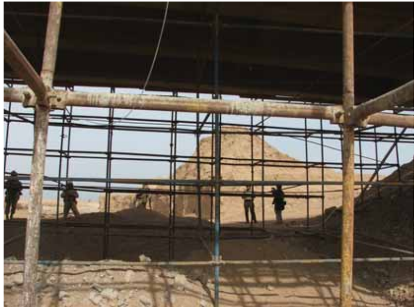
SIGIR's inspection of the Mujarrah Canal Bridge found some faulty construction, but overall the work met most design specifications.
