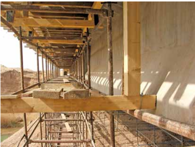
Falsework for forming concrete deck overhang for the Mujarrah Bridge.
