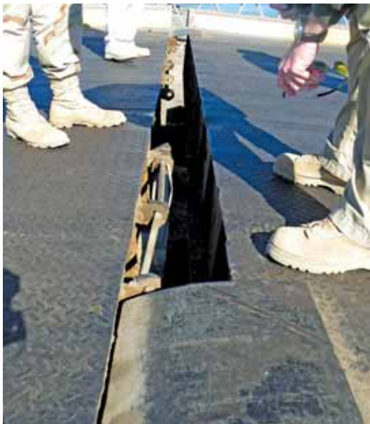
RORO Berth 22 deck hinges.
