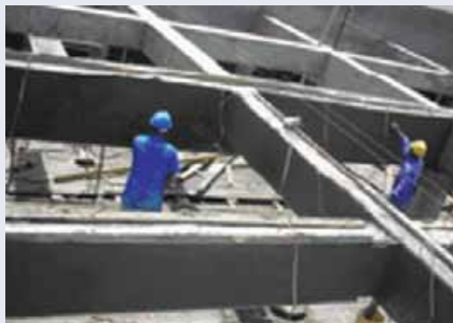
Workers build stalls in the new al-Kut Meat Market in Wassit province. (USACE photo)
