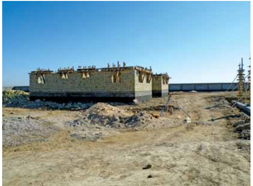
Ongoing construction of the physician's residence at the Missan Surgical Hospital.
