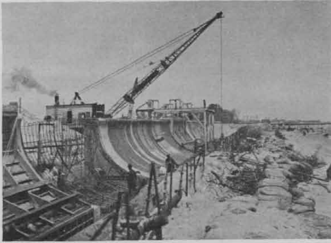
Constructing the new sea wall.
