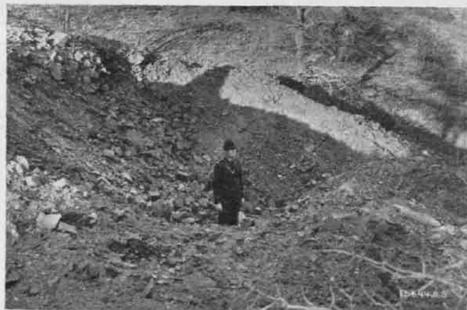
Crater made in the granite rock of Wichita Range by explosion of 2,000 pound bomb. Dimensions: 12 feet deep by 31 feet in diameter. Bomb dropped from 15,000 ft. altitude.
