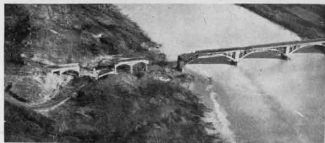
View of Pedee River bridge showing extent of damage after a direct hit by a 1100 pound bomb.
