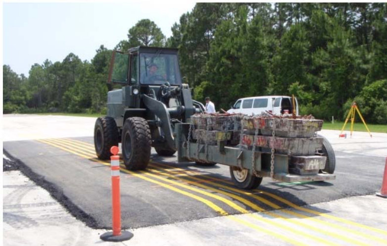
FIGURE 4 F-15E load cart testing helped evaluate rutting resistance of test sections.
