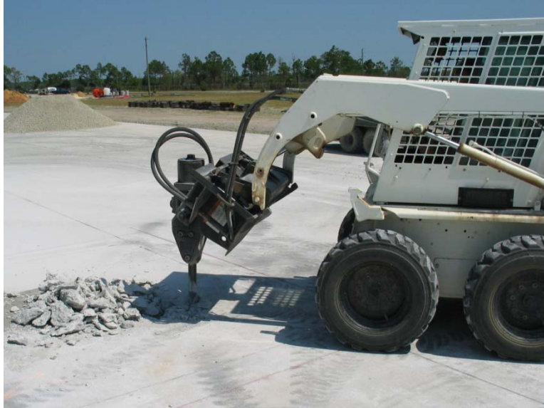
Figure 3. Hydraulic Breaker on Wheeled Skid Steer Loader.
