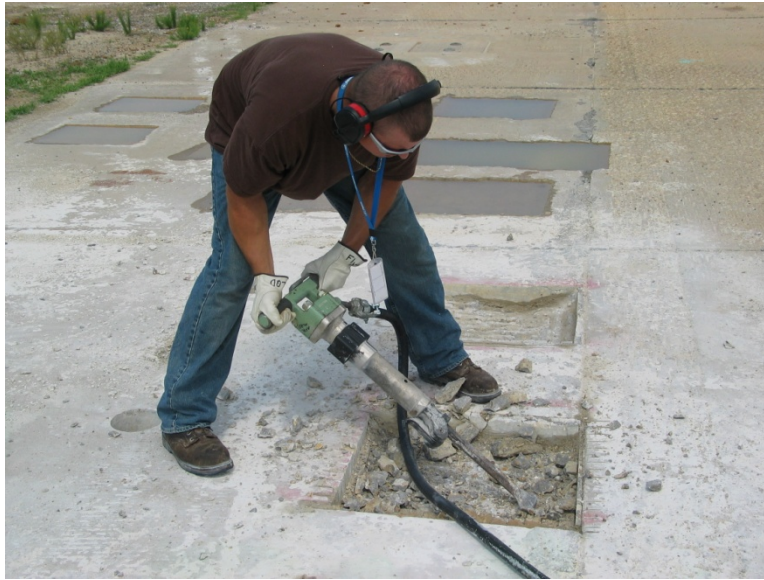
Figure 1. 30-lb Jackhammer Used to Prepare Spalls.
