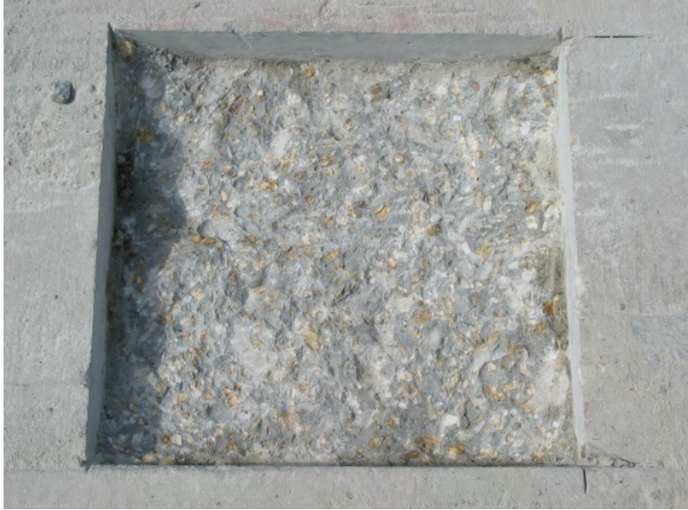
Figure 2. Photo of Completed Excavation using 30-lb Jackhammer.
