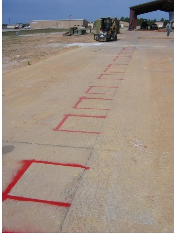
Figure 11. Layout of Spall Locations before Excavation
