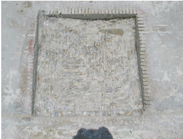
Figure 10. Saw-cut Excavation (3/4-inch Spacing) after Removal of Debris.
