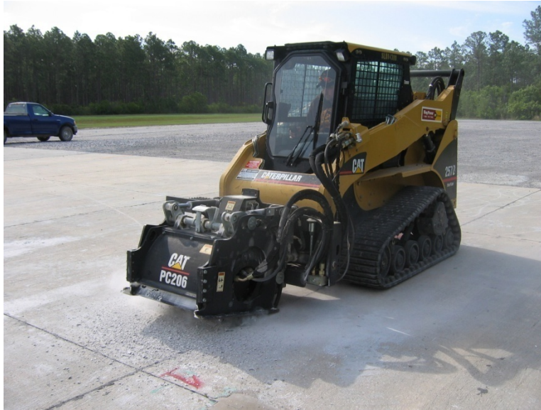
Figure 5. Cold Planer on Skid Steer Loader.
