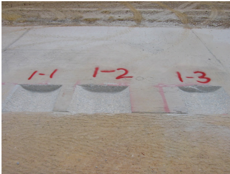
Figure 7. Excavations Prepared with Cold Planer.
