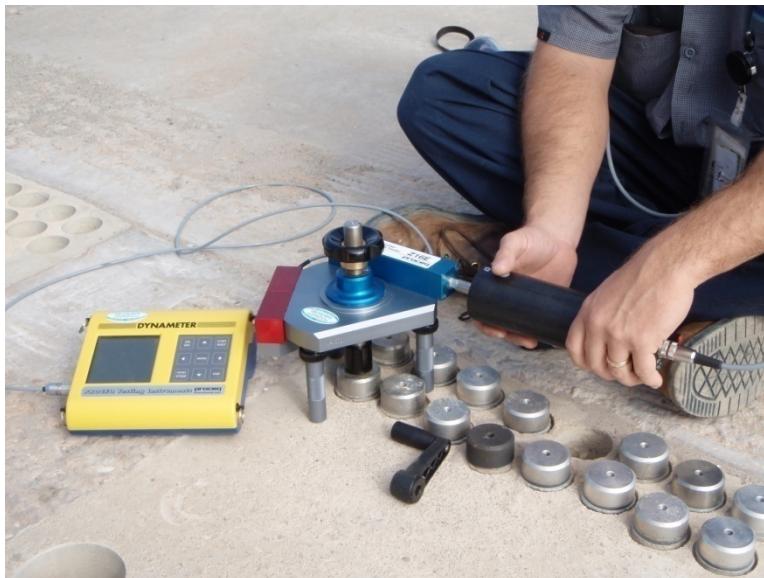
Figure 19. Photograph of In-Situ Tensile Pull-off Test in Progress.
