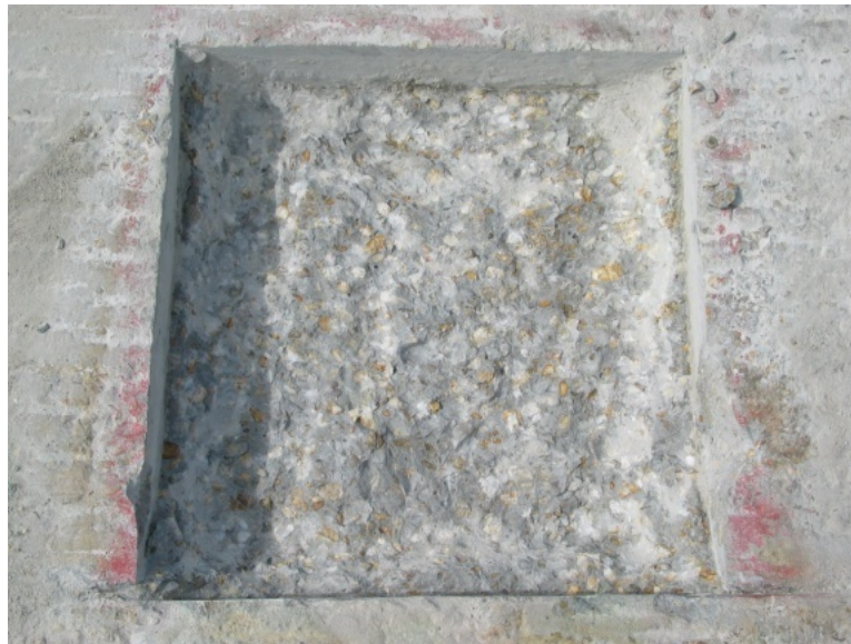
Figure 4. Hole Excavated using Hydraulic Breaker.
