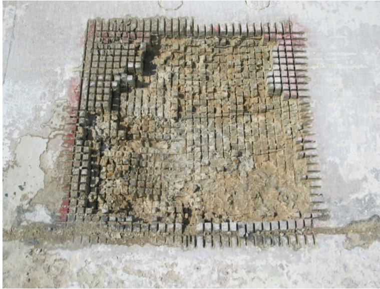
Figure 9. Saw-cut Excavation (3/4-inch Spacing) Prior to Removal of Debris.
