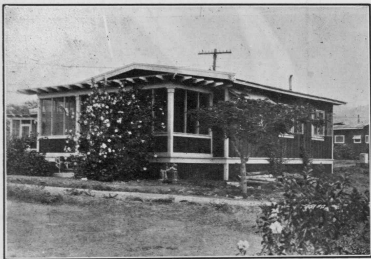
BUNGALOW TYPE OF QUARTERS, FORT SHAFTER
