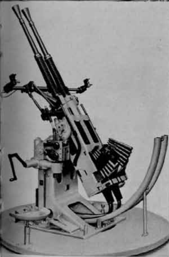
6. 25 mm. A.A. Gun, Twin Mount. Rate of fire: 300 rds. per minute.
