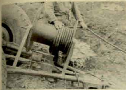
Cable rack in action.
