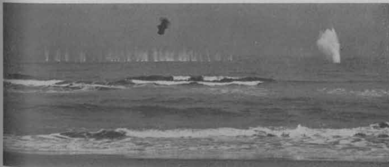
A rarely photographed action: the ricochet, burst, and subsequent fragmentation of a point detonating H.E. projectile. The tall column of water on the right side of the picture is the splash, the black smoke puff is the explosion, and the spray beneath that is caused by the pieces of metal from the projectile itself.
