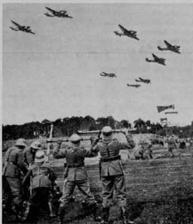
German Machine Gun in Action. Note one-meter range finders and method of support.
