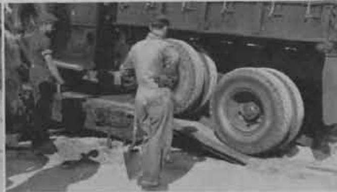
Left: The ramp ready for use with short metal ramps of boiler plate in place. Note hole in roadbed to receive the short ladder on side of car. A plank, laid cross grain, acts as a cushion between car and rails. Right: A prime mover starts across the ramp.
