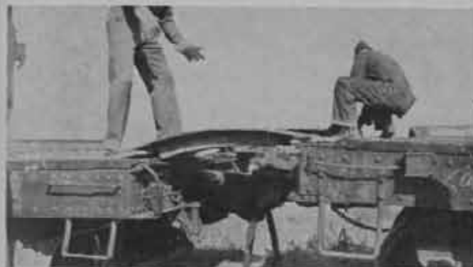
Left: Putting the crossovers in place. Right: Illustrating one method of blocking and snubbing. Notice the crossovers.
