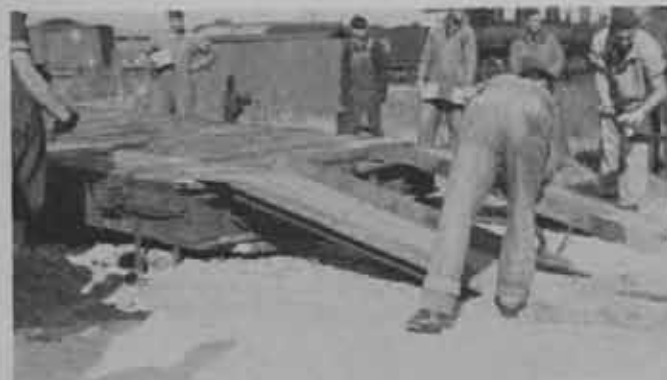
Left: The ramp ready for use with short metal ramps of boiler plate in place. Note hole in roadbed to receive the short ladder on side of car. A plank, laid cross grain, acts as a cushion between car and rails. Right: A prime mover starts across the ramp.
