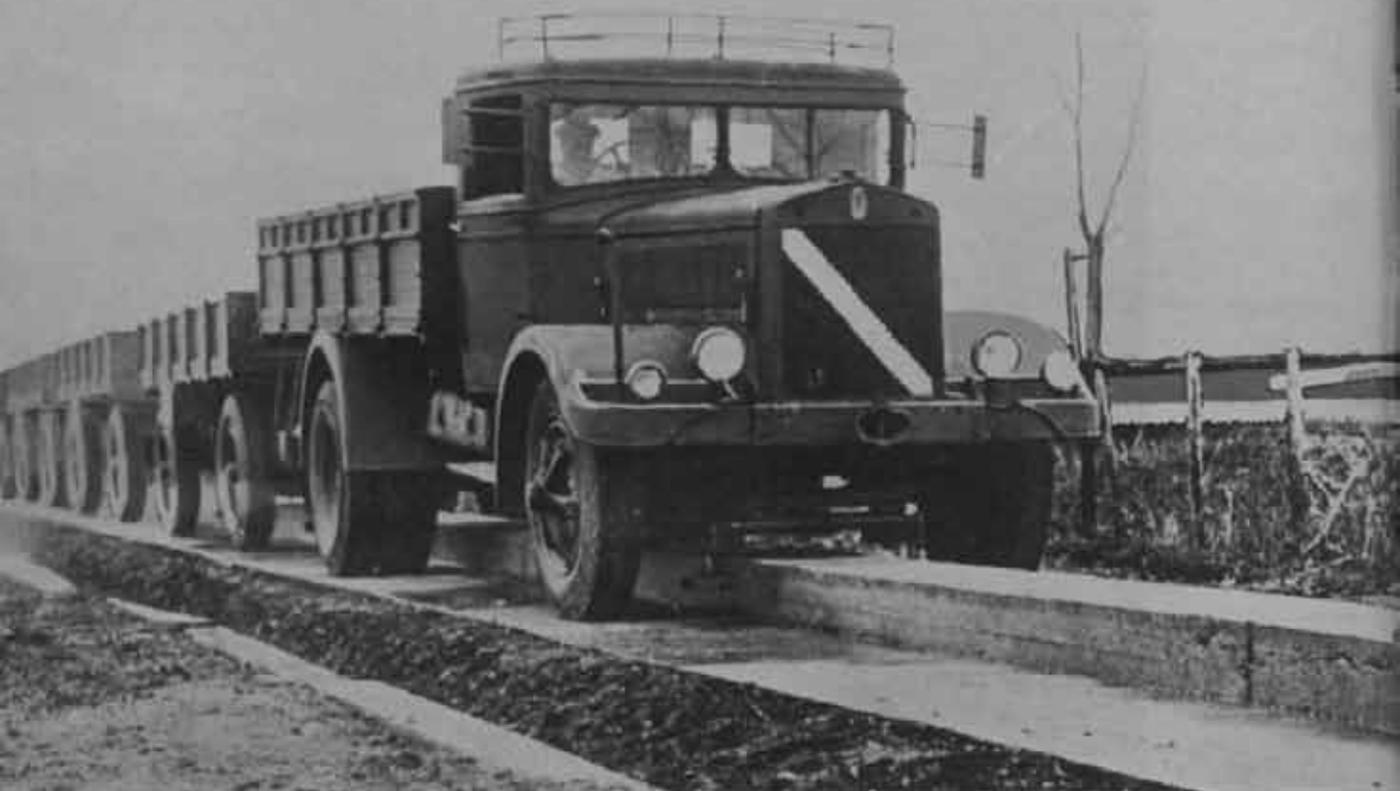
↑ *This experimental military road, recently tested near Rome is designed to permit a truck to tow a string of trailers*
