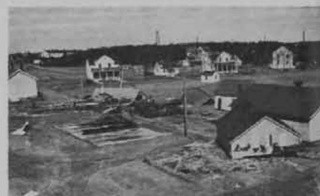
Utility area at Fort Rodman, Massachusetts, after the hurricane.
