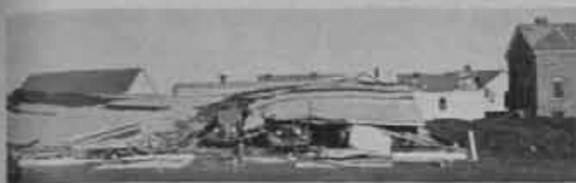
Ruins of a garage at Fort H. G. Wright, New York, after the hurricane.
