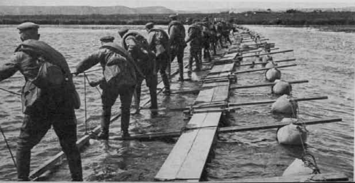
• Left: A bridge made of rafts. In a few minutes, Soviet infantrymen crossed the river.
