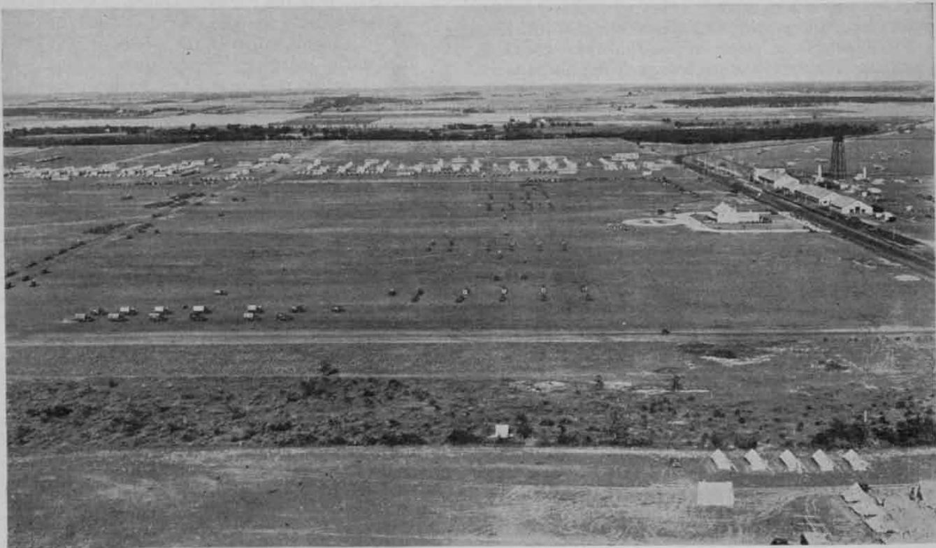
Camp Ripley, the New Camp of the Minnesota National Guard at Little Falls, Minnesota.
