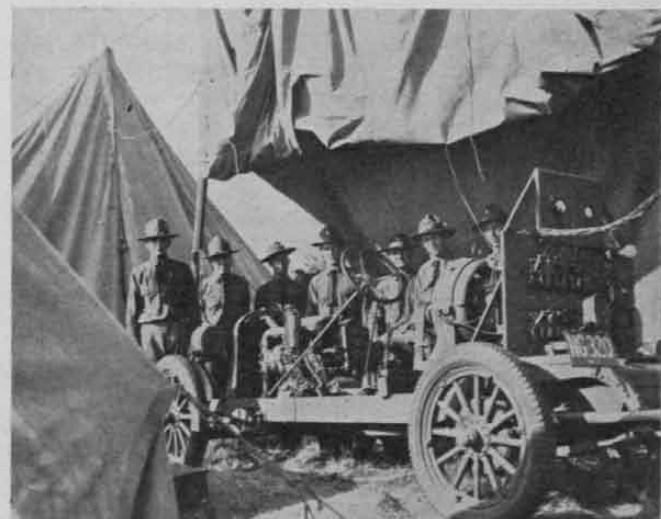
Generator and Electricians Who Furnished Tent Lights to 1st Corps of Cadets at Peter's Pond, South Sandwich, Mass., 1932.
