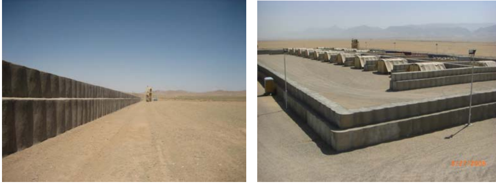
Figure 4. Ammunition Supply Points in Herat (left) and Mazar-e-Sharif (right) Lack Security Fencing Around the Perimeter
