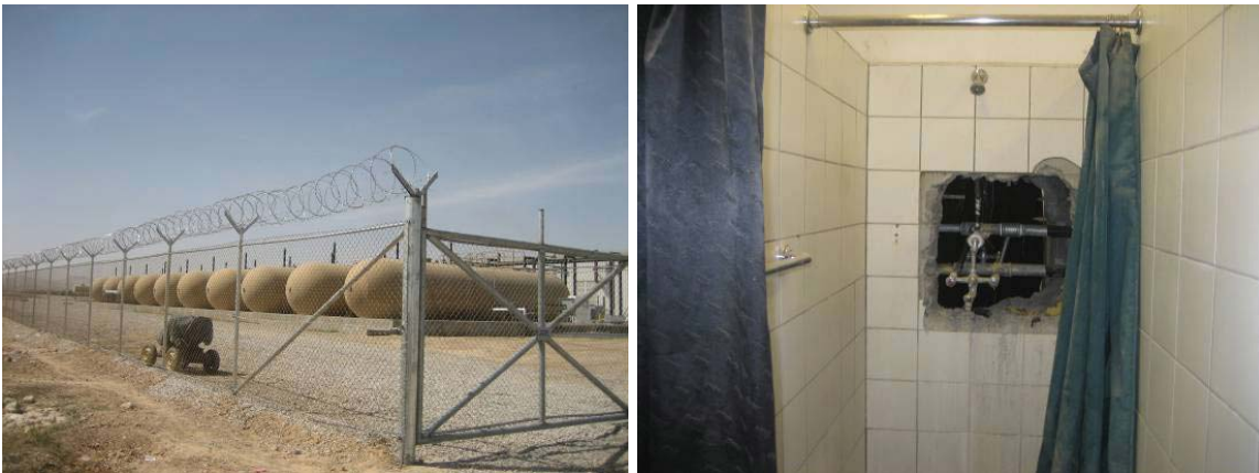
Figure E-8. Fuel Storage Tanks (left) and Frozen Pipes (right) at MeS
