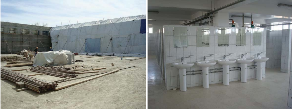
Figure E-3. NMAA Gym (left) and Latrine (right)
