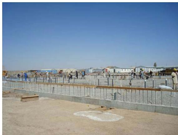
Figure E-6. Kandahar Hospital Addition Under Construction
